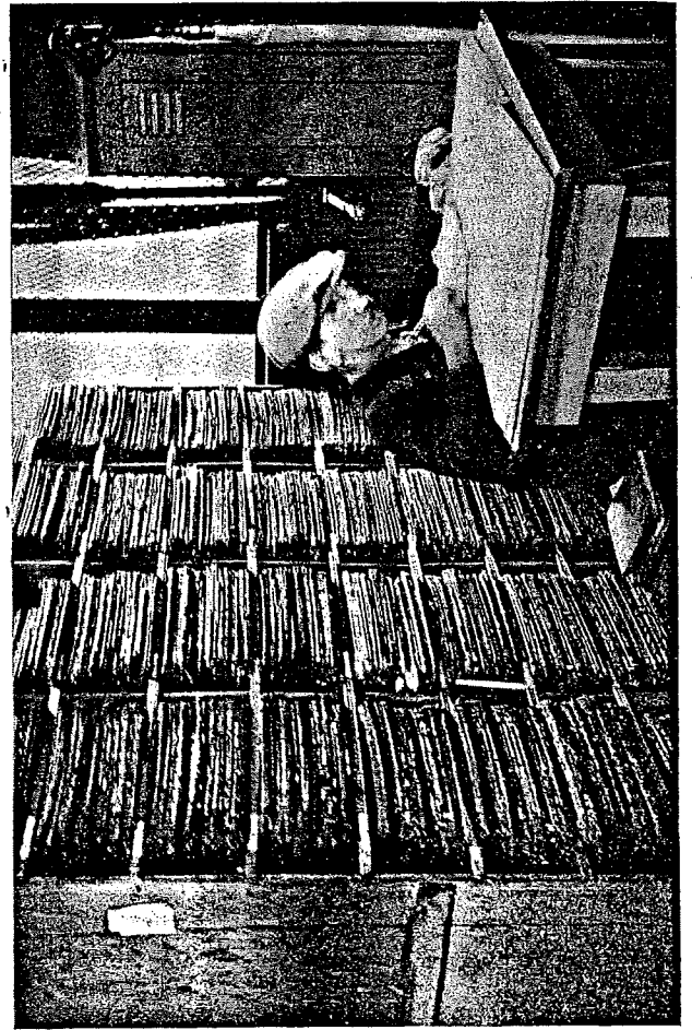
Interior of card room showing method of storing boiler cards
