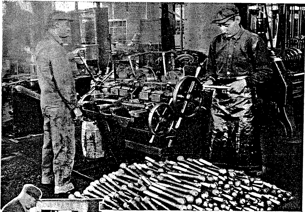
(Above)—Machine set up for threading flexible staybolts
