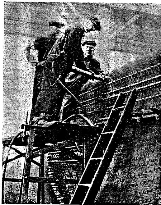
On receipt of the boiler, the odd rivets, which can not be fitted on the bull riveters, are driven by hand
