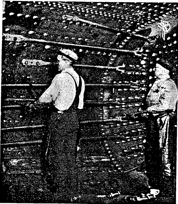
In fitting backhead braces, two men work on the inside of the boiler and one on the outside applying assembly bolts
