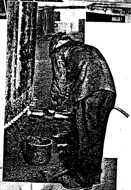
Inserting odd rivets in the barrel
