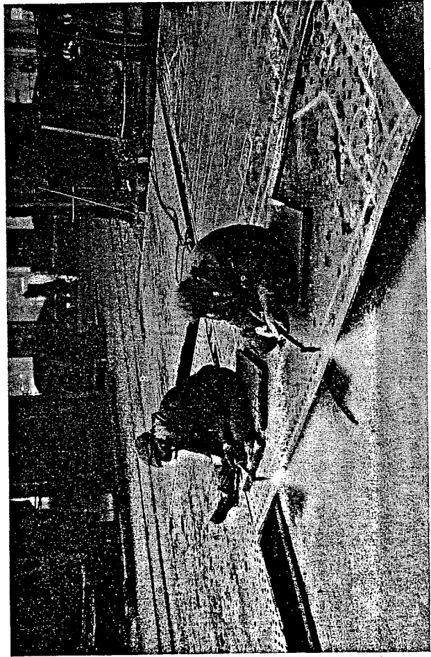
Cutting the edges of a roof top and side sheet before planing
