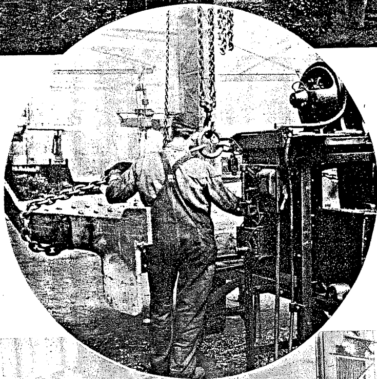
(Left) — Drilling throat sheet rivet holes on a horizontal drill
