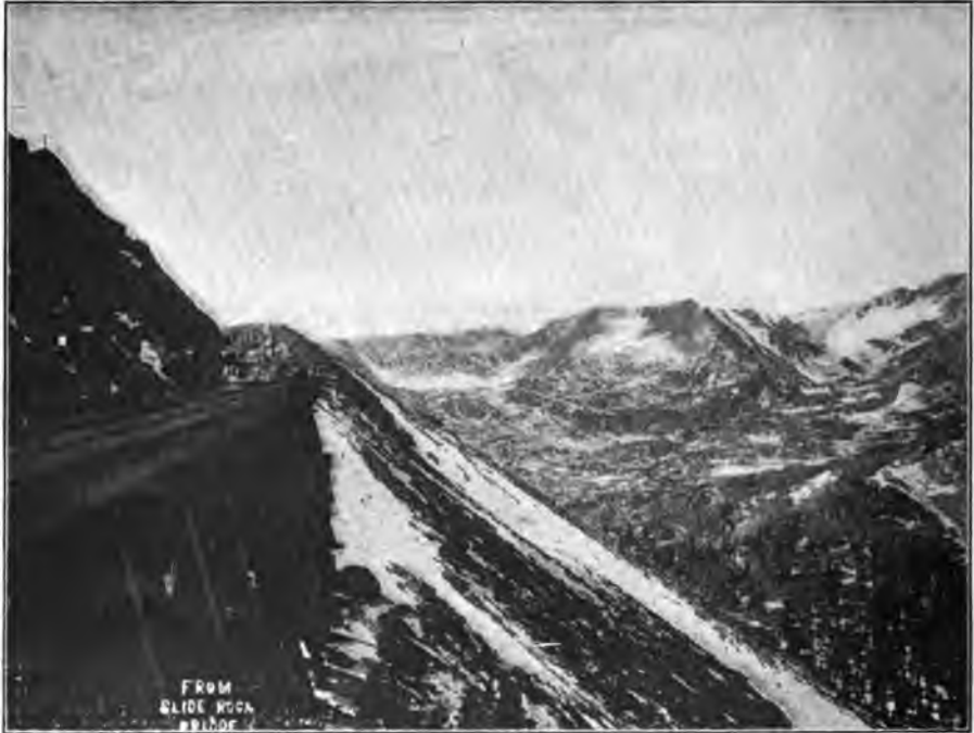
SOME OF THE DIFFICULTIES OF CONSTRUCTION, MOFFET ROAD, COL.—F. J. FRANCIS, PHOT'R.
