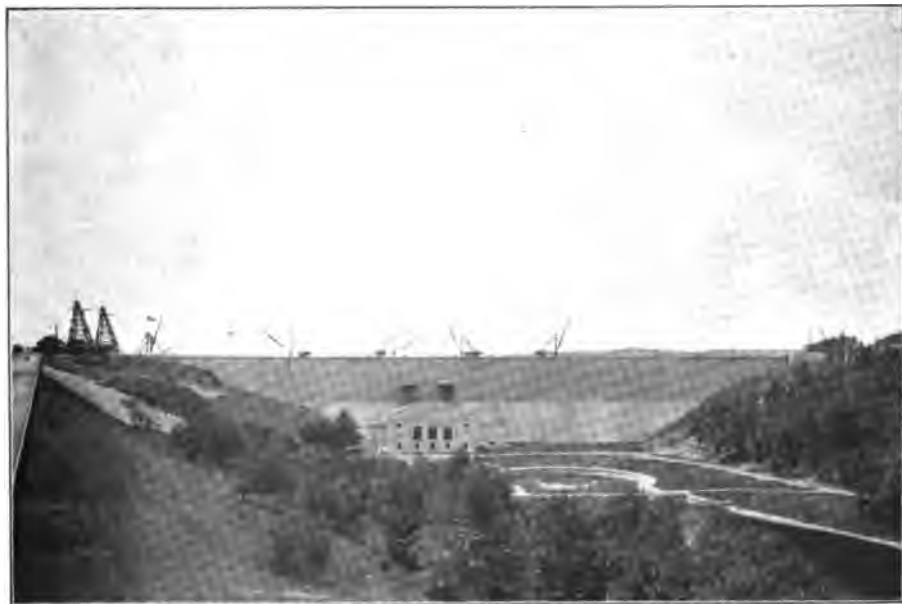
VIEW OF THE FACE OF THE WACHUSETT DAM, SPILLWAY AND GATEHOUSE COMPLETE, WITH TROLLEY DERRICKS WHICH WERE USED IN CONSTRUCTION STILL IN PLACE.
