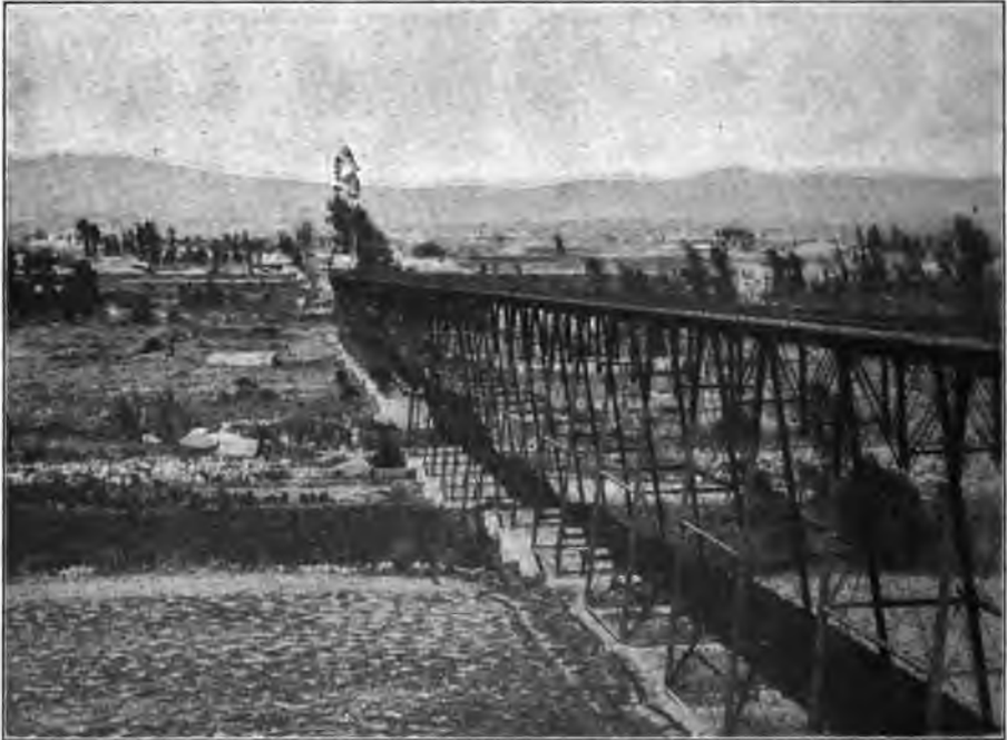
AREQUIPA RAILROAD BRIDGE 6,000 FEET LONG, WITH RAILING AND WALK ON EITHER SIDE OF TRACK.
