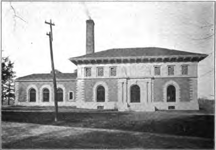
PUMPING STATION, BOSTON WATER SYSTEM.
