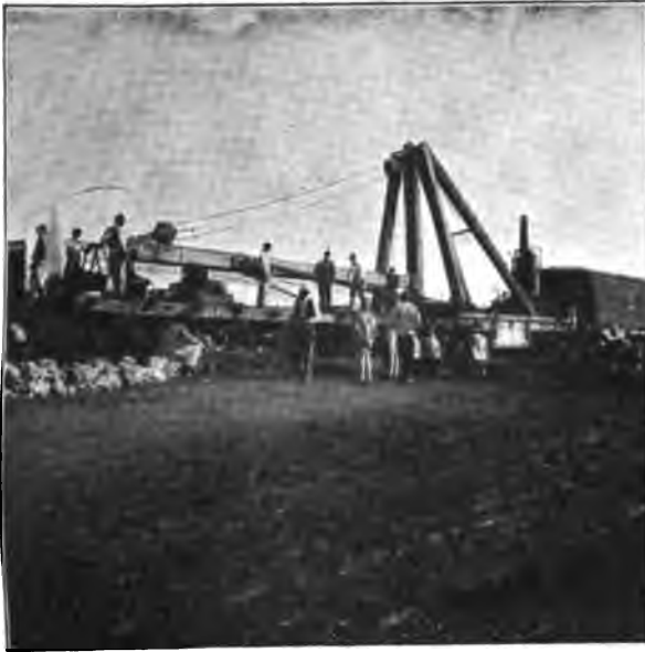
CUBA RAILROAD DERRICK CAR.
