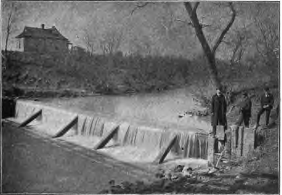
SULPHUR CREEK DAM, FRANKLIN JUNCTION, MO.—COURTESY J. S. CARLISLE, DIV. 556.
