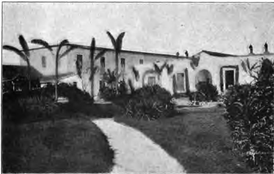
HOTEL CAMAGUEY GARDENS, CAMAGUEY, CUBA.—COURTESY P. O. RICKMAN.
