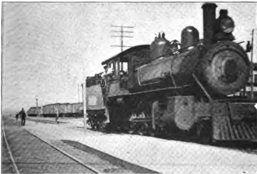
NEWTON & ISON TRAIN ORDER CRANE IN POSITION.
