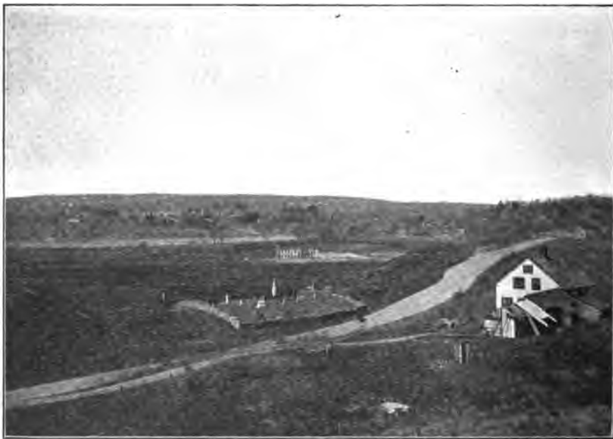
NECESSARY DESTRUCTION OR REMOVAL OF STRUCTURES.
