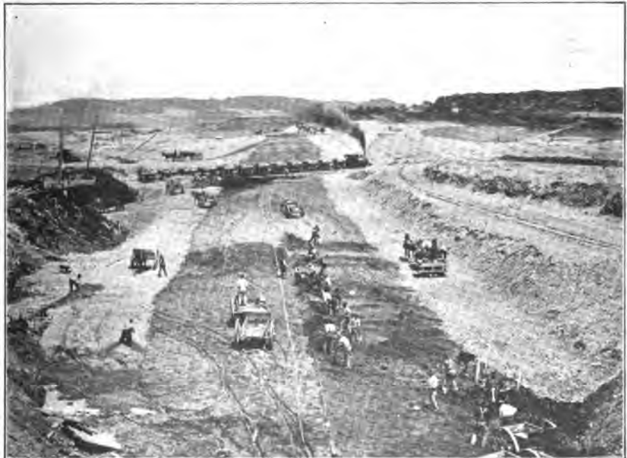
THE GREAT WORK OF LEVELING THE BASIN ABOVE THE WACHUSETT DAM.
