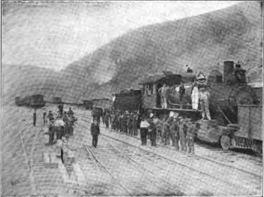
BALTIMORE & OHIO MAKING A NEW YARD NEAR PITTSBURG, PA.—Full Brotherhood crew manning the engine with Bro. J. F. Bainter, of Div. 379, at the throttle, and construction gang.—Courtesy J. F. B.
