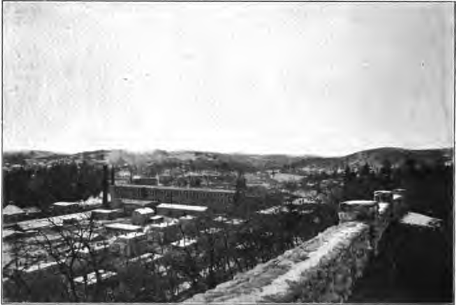
CLINTON, MASS., LOOKING TOWARDS LOCATION OF DAM.
