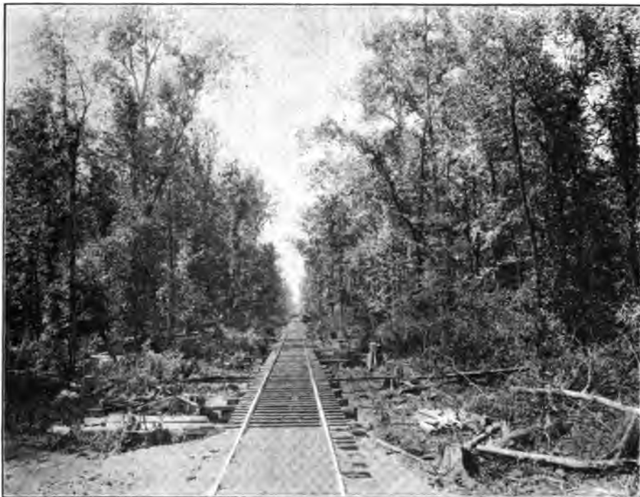
DEERING & SOUTHWESTERN RY., CONSTRUCTION THROUGH SINK LANDS IN MISSOURI.
