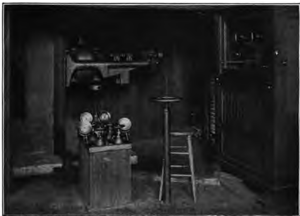
FIG. 88.—A center of control. Valves controlling water circulation in friction brakes, the traction dynamometer and scale case.
