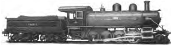
COMPOUND CONSOLIDATION LOCOMOTIVE For the Bavarian State Railways
