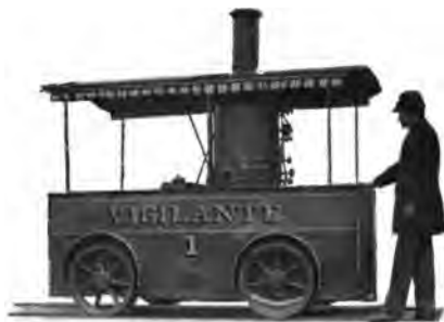
STEAM INSPECTION CAR
