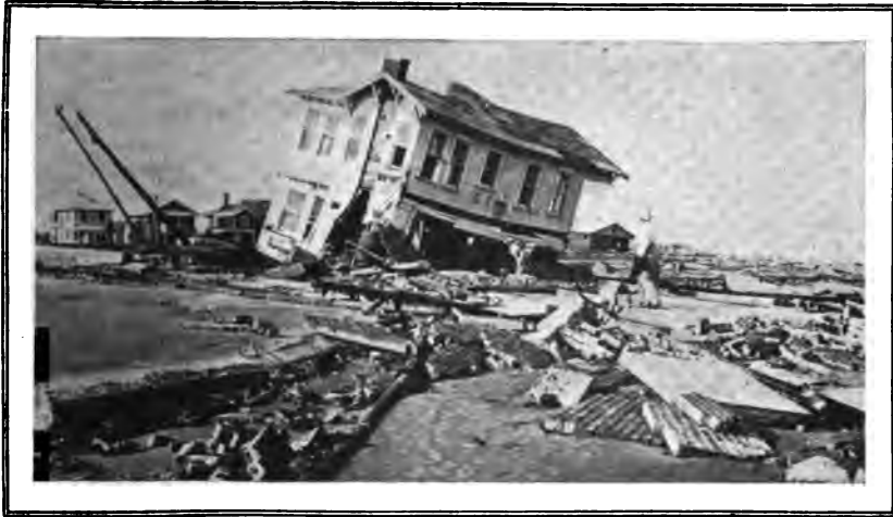
THE BOULEVARD AND EIGHTH STREET
