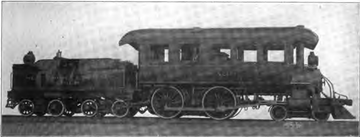
Fig. 55. Eight-Wheel (4—4—0) Inspection Locomotive. Built by the American Locomotive Co. for the New York Central Lines. Cylinders 15 in. x 24 in., Working Steam Pressure 200 lbs. per sq. in., Heating Surface 1,044.75 sq. ft., Diameter of Drivers 62 in., Weight on Drivers 66,500 lbs., Total Weight 99,500 lbs.
