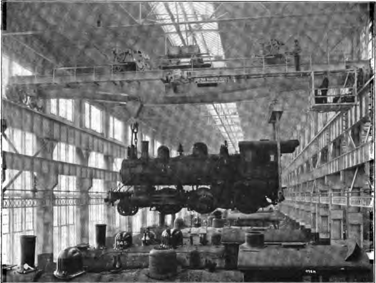
120-Ton Crane Installed in New Railroad Shops of The Grand Trunk Ry. System at Battle Creek, Mich. Span 67' 6".
