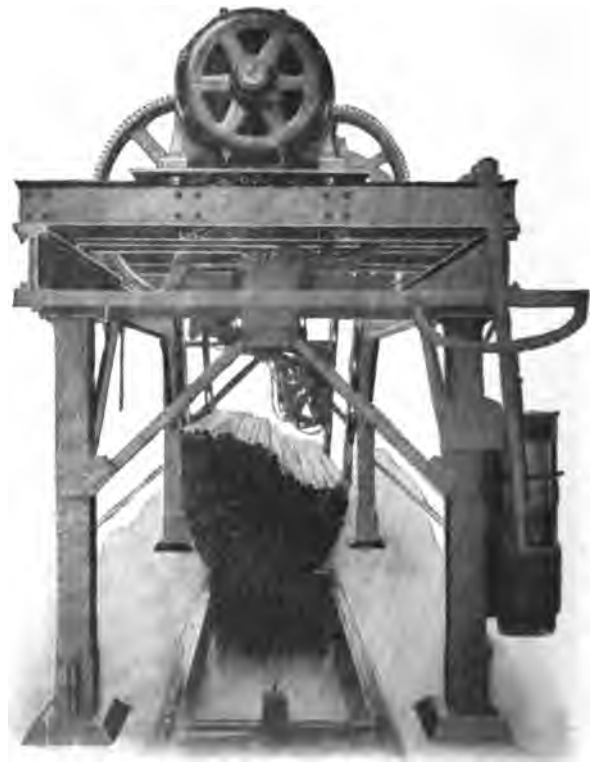
Fig. 5147. Flue Cleaning Machine. Joseph T. Ryerson & Son.
