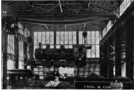
Westinghouse Motors Operating Traveling Crane.
