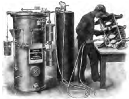
Fig. 5265. Oxy-Acetylene Welding Plant in Operation. The Davis-Bournonville Co.
