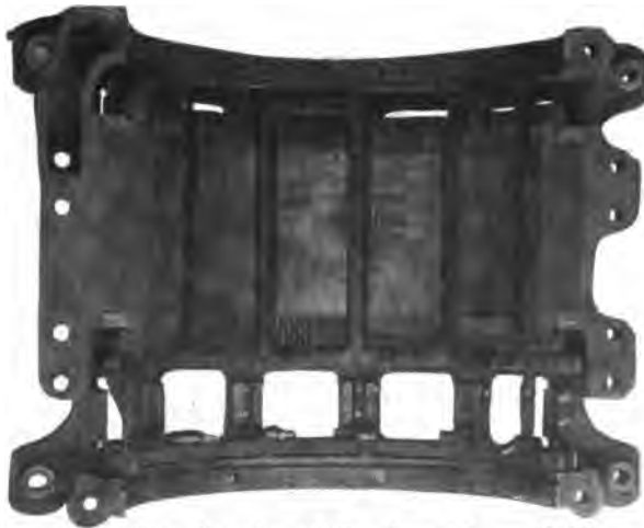
Fig. 4698. Interior of Gearless Motor Field. Westinghouse A. C. Electric Locomotive.
