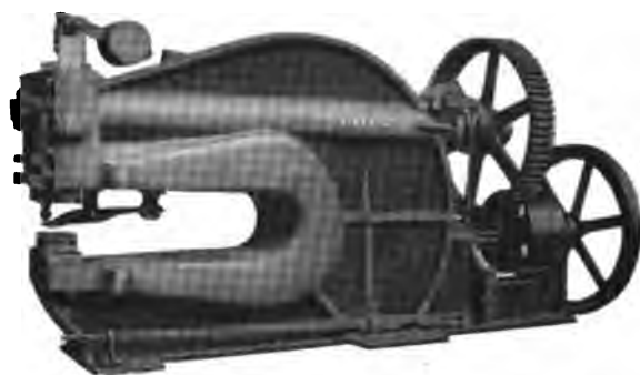
Fig. 5231. Solid Frame Punch, Equipped with Plain Jaw. Joseph T. Ryerson & Son.
