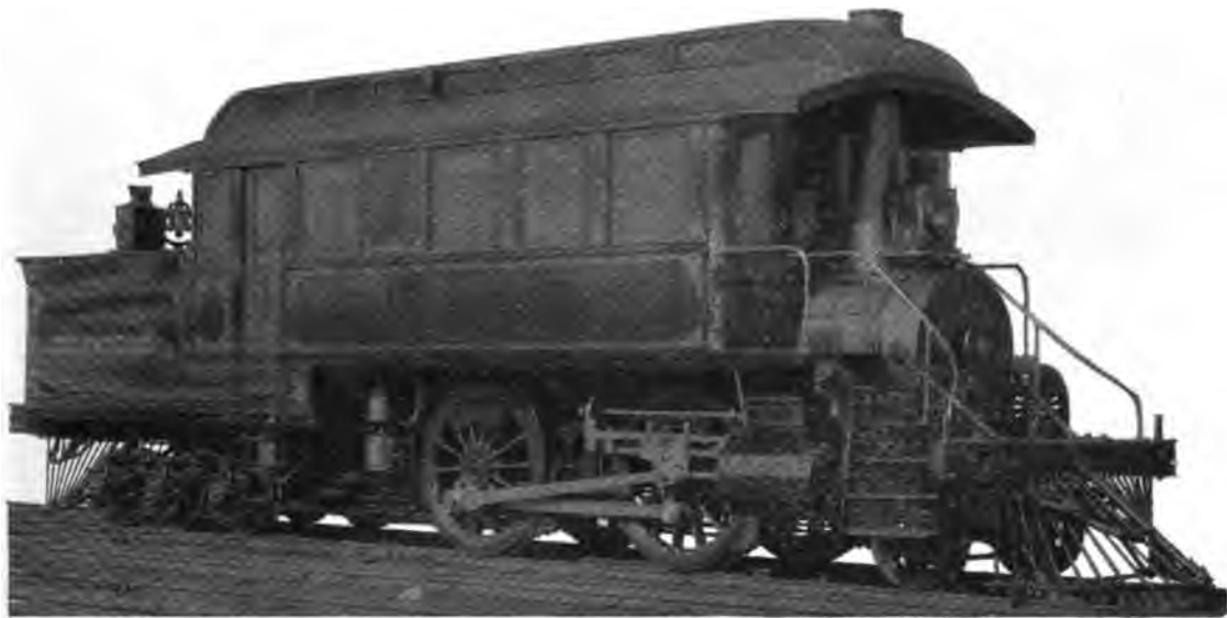
Fig. 32. Four-Coupled Double Ender (2-4-6) Inspection Locomotive. Built by the American Locomotive Co. for the Adirondack & St. Lawrence. Cylinders 16 in. x 22 in., Working Steam Pressure 160 lbs. per sq. in., Diameter of Drivers 60 in., Weight on Drivers 57,000 lbs., Total Weight 134,000 lbs.
