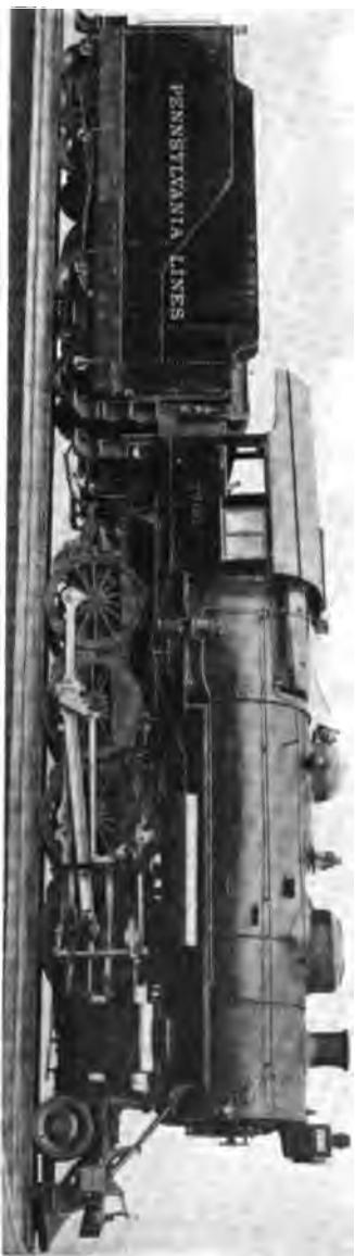
FIG. 19.—Freight locomotive. 2-8-0 type (Consolidation).
