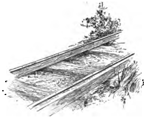
TRACK WITH WOODEN STRINGERS, SURFACED WITH STRAPS OF IRON
