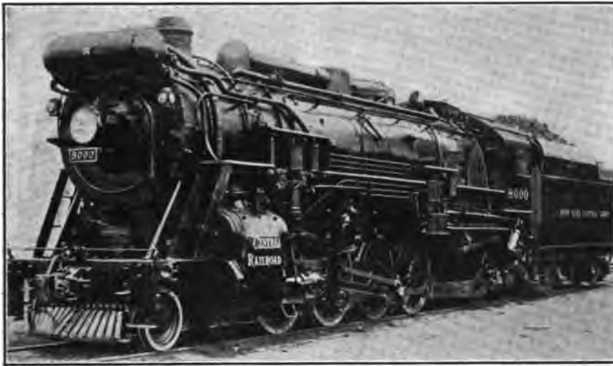
VIEW OF LOCOMOTIVE NO. 8000, MICHIGAN CENTRAL, SHOWING FEED-WATER HEATER LOCATION IN FRONT OF THROTTLE AND STACK
