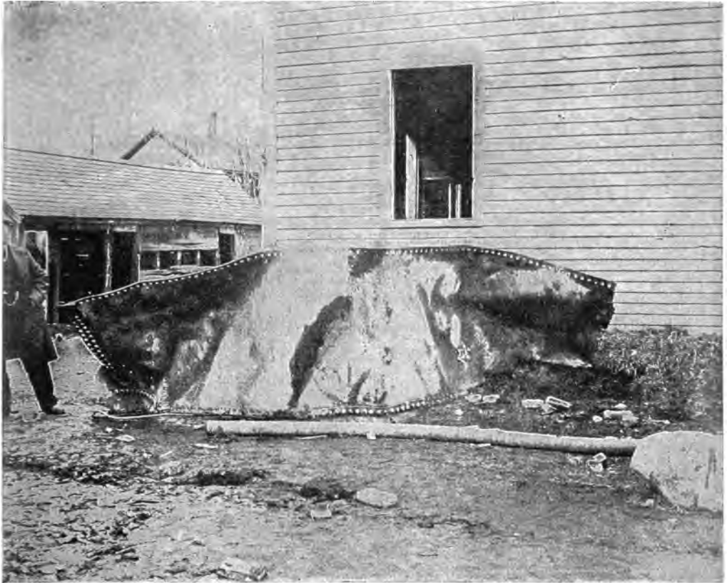
FIG. 4. — A SECTION OF THE EXPLODED BOILER.
