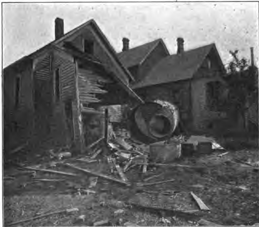
BOILER EXPLOSION AT OWOSSO, MICHIGAN.
