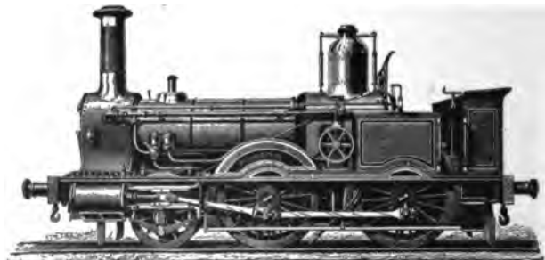
FIG. 79.—BEATTIE'S 4-COUPLED TANK ENGINE, L. & S.W.R., 1857
