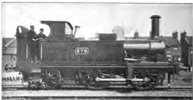
FIG. 135.—4-COUPLED-IN-FRONT PASSENGER TANK ENGINE, G.W.R.
