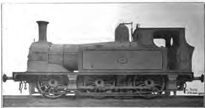
FIG. 126.—"No. 143," TAFF VALE RAILWAY INCLINE TANK LOCOMOTIVE
