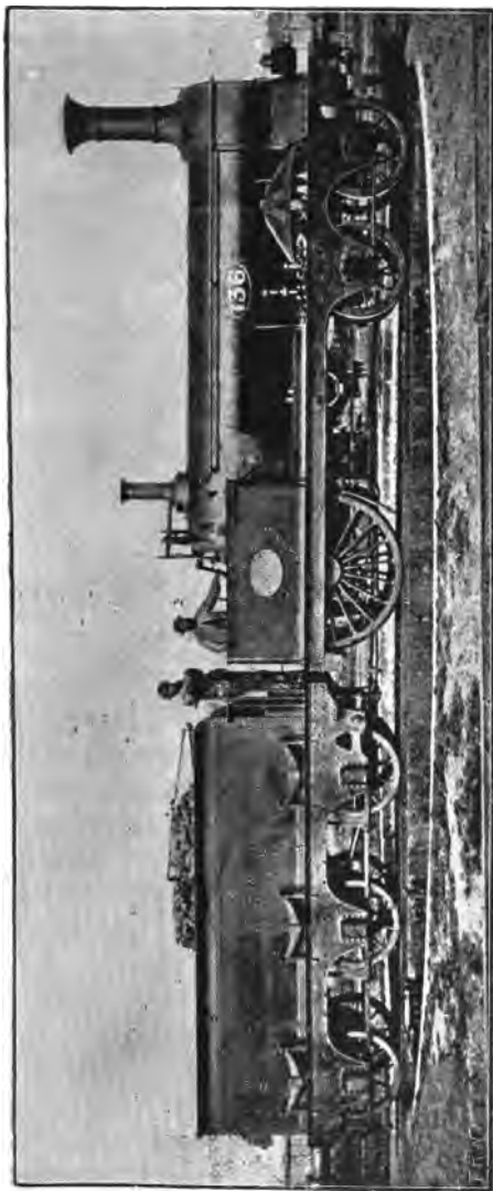
FIG. 61.—THE "FOLKESTONE," A LOCOMOTIVE ON CRAMPTON'S SYSTEM. BUILT FOR THE S.E.R., 1851
