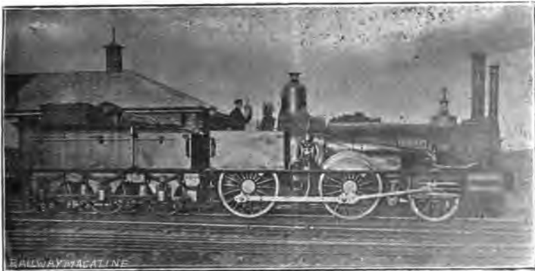
Fig. 76.—THE "DANE," L. & S.W.R., FITTED WITH BEATTIE'S PATENT APPARATUS FOR BURNING COAL
