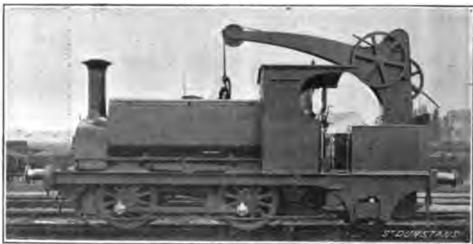
FIG. 89.—LOCOMOTIVE AND TRAVELLING CRANE, N.L.R.
