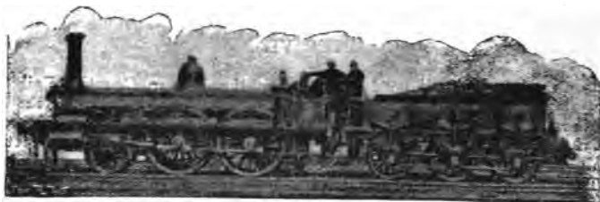
FIG. 35.—STEPHENSON'S "LONG-BOILER" GOODS ENGINE, EASTERN COUNTIES RAILWAY
