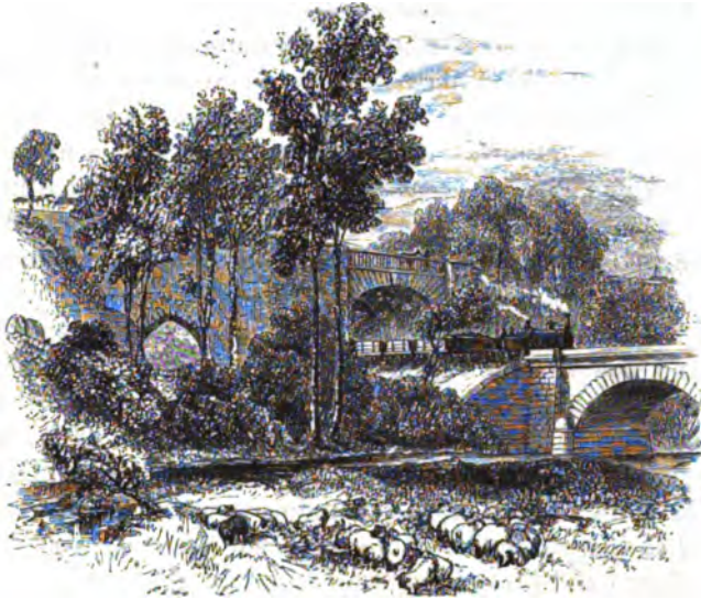
BULL BRIDGE, NEAR AMBERGATE.
