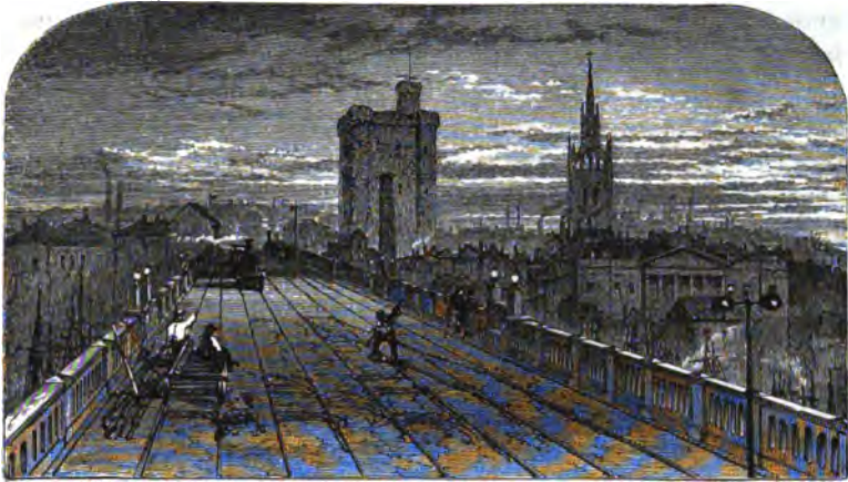
NEWCASTLE, FROM THE HIGH-LEVEL BRIDGE. [By R. P. Letch.]
