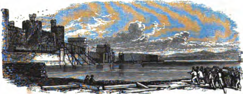
CONWAY BRIDGE—FLOATING THE FIRST TUBE.
