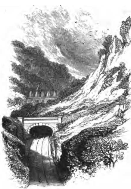
LAND-SLIP ON NORTH MIDLAND LINE, NEAR AMBERGATE.
