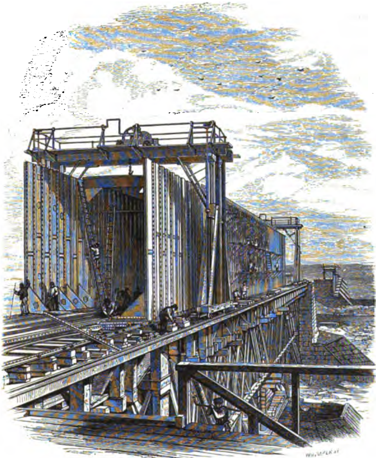
ERECTION OF MAIN CENTRAL TUBE.
