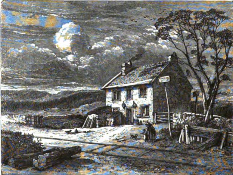
HIGH-STREET HOUSE, WYLAM. [By R. P. Leitch.]
