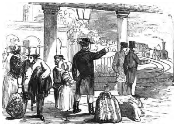
INTERIOR OF A STATION.
