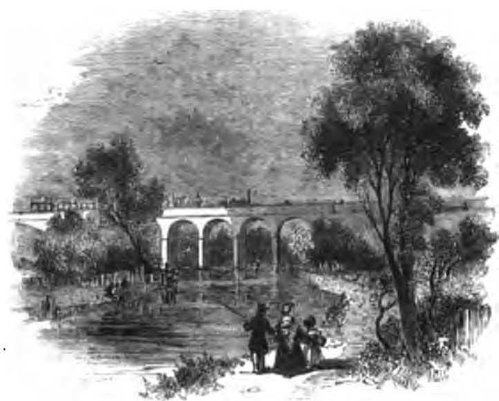
VIADUCT, NEAR WATFORD, BIRMINGHAM RAIL-ROAD.
