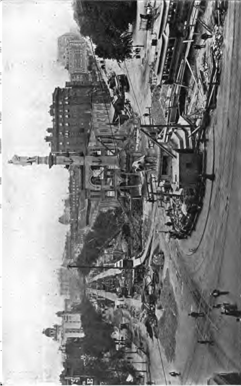
FIG. 24. NEW YORK SUBWAY IN COURSE OF CONSTRUCTION. CAR TRAFFIC MAINTAINED
