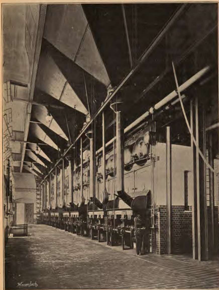
FIG. 17. BOILER-ROOM, LONDON UNITED TRAMWAYS CO.'S POWER HOUSE AT CHISWICK, FITTED WITH VICARS' AUTOMATIC STOKERS
