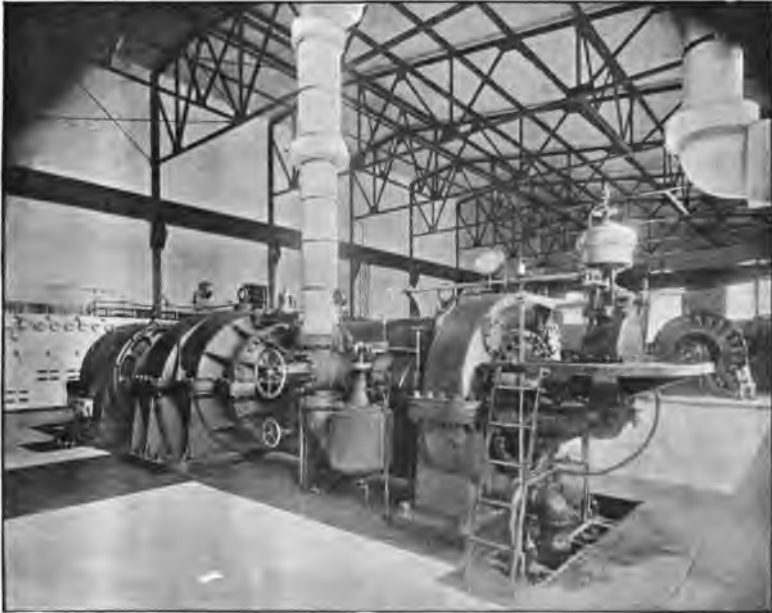
FIG. 9. A 2,000 H.P. WESTINGHOUSE STEAM TURBINE, RESEMBLING THE TURBO-GENERATORS (EACH OF 7,500 H.P.) IN THE CHELSEA POWER HOUSE.
