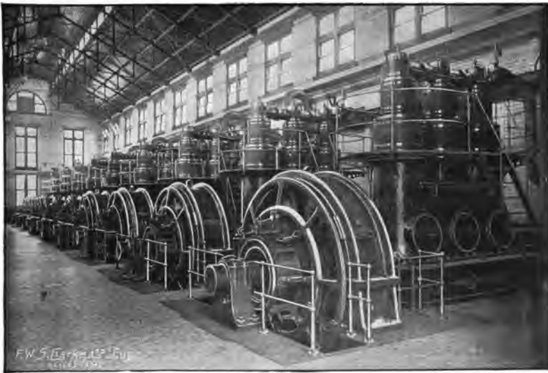
FIG. 2. NINE WILLANS-SIEMENS DYNAMO SETS FOR ELECTRIC TRACTION, 700 H.P. EACH.
