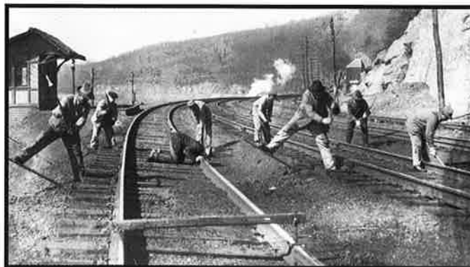
Workmen using new method of leveling tracks October 28, 1918. Penn Central Corporation Collection of Pennsylvania Railroad Negatives. Courtesy of Hagley Museum & Library, Wilmington, Delaware
