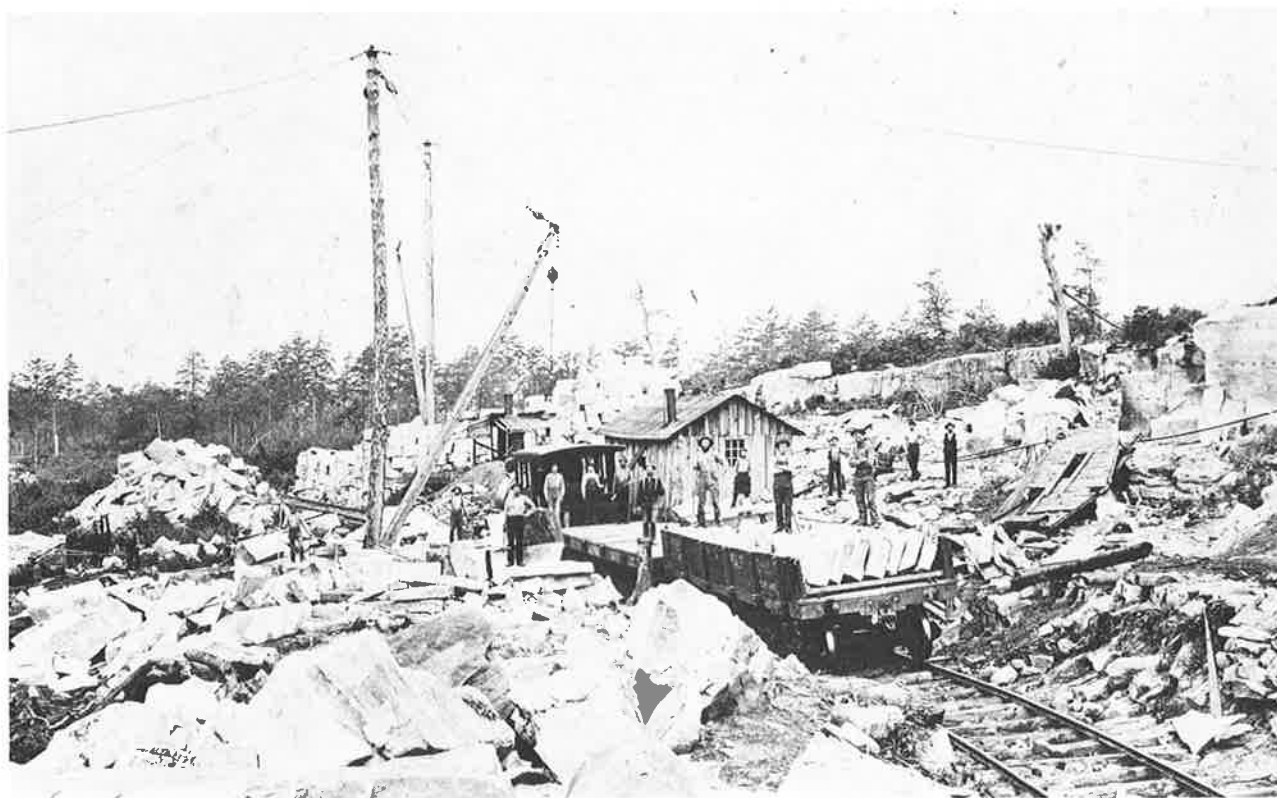
The reason for the Bare Rock Railroad was this quarry. A Baltimore and Ohio low sided gondola has been loaded with cut rock. The small building by the locomotive housed a steam engine for operating the crane. A similar crane in the rear is served by a vertical boiler and steam engine unprotected by a building. This is a very typical view of rock quarry operation and its railroad.
