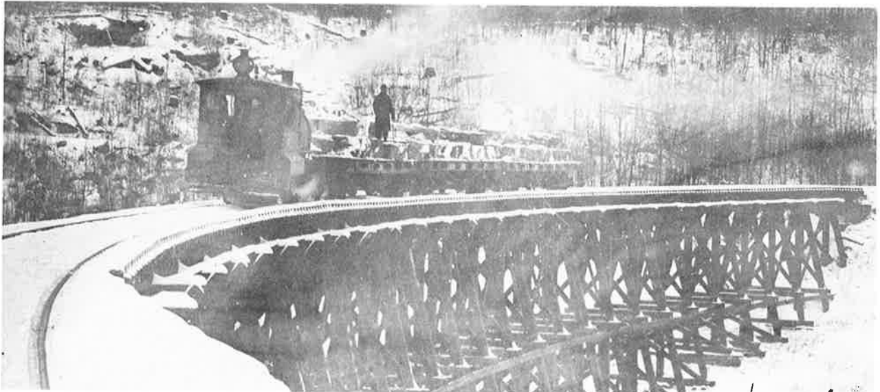
A saddle tank switcher crosses over the trestle of the Bloom Run RR as it brings three cars of cut stone down the mountain.
