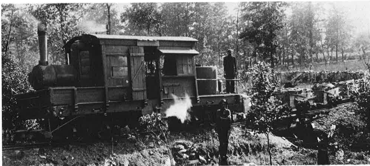
The General Refractory's clay train swings around a curve on its five mile trip to the brick yard at West Decatur, Clearfield County. The "box car" Climax had a maximum speed of seven miles an hour which was just about right for the little clay cars.
