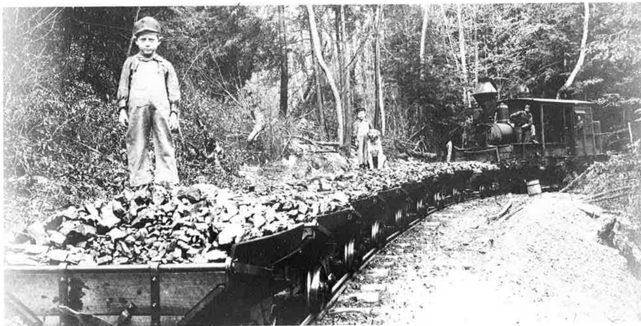
A. B. Lansberry Coal Co's narrow gauge train ran from mine to New York Central coal tipple reload point. Each of the 9 or 10 cars held about 1-1½ tons. The "box car" Climax was popular with small narrow gauge coal, clay, and logging railroads because of its power and winter protection for the crew.
