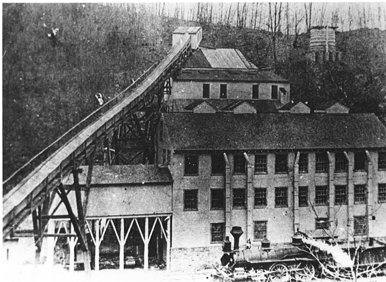
Near the Susquehanna River squeezed between two mountains was the iron mine and concentrating mill of the Champion Iron and Separating Company, an unsuccessful company which for ten years from about 1902 to 1912 operated its mill and a 4½ mile railroad to reach it. This picture shows their only 4-4-0 and the facilities photographed from one hillside looking across the narrow hollow toward the opposite hillside. This was the only line-haul private iron ore carrying railroad in Pennsylvania which did not incorporate as a common carrier.
