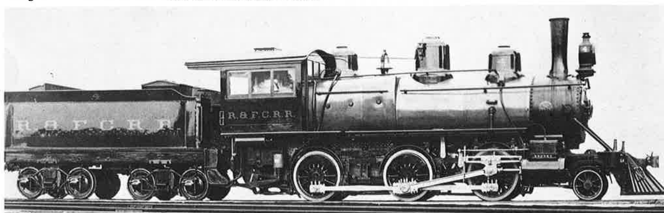
Reynoldsville and Falls Creek #4 built in 1897 and similar to a group of locomotives built about the same time by Brooks for the Great Northern Railroad. This engine spent its final days on the Arcade and Attica R.R., No. 8, in New York State.
