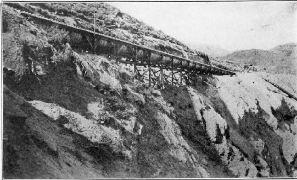
FIG. 1.—DOUBLE-CHANNEL FLUME IN THE PAYETTE VALLEY.
