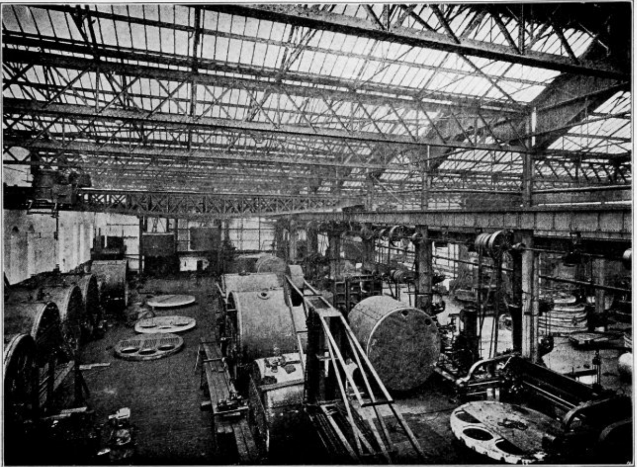
BUILDING AND FLANGING BAYS OF ROWAN'S BOILER SHOP.
