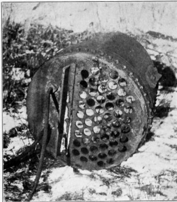
FIG. 3.—FRONT TUBE SHEET AND PORTION OF SHELL.
