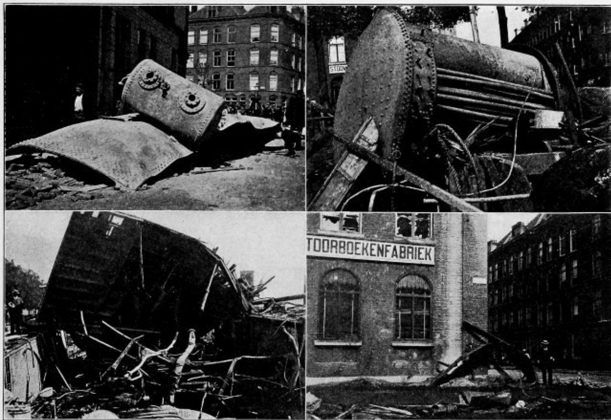
FIG. 1.—DOME AND FLATTENED SHELL. FIG. 3.—DECK OF THE SHIP AFTER EXPLOSION.
