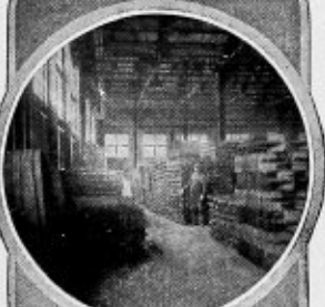
Boiler Lugs and Hangers
