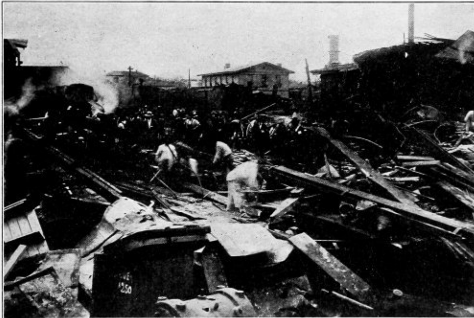
WRECKAGE CAUSED BY A LOCOMOTIVE BOILER EXPLOSION ON THE SOUTHERN PACIFIC
