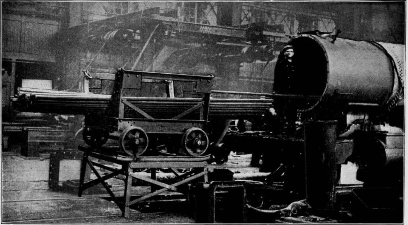
FIG. 2.—REMOVING TUBES FROM THE BOILER AND LOADING ON THE FLUE CAR IN THE ERECTING SHOP
