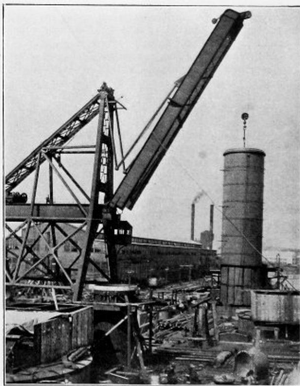
PLACING A 38-TON SMOKESTACK ON BOARD A BATTLESHIP
