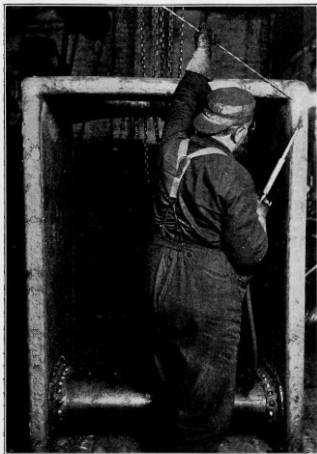
FIG. 3.—WELDING THE MUD-RING
