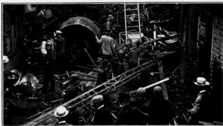
BOILER EXPLOSION, LAKEPORT STEAM LAUNDRY, LACONIA, N. H. 1 KILLED; 7 INJURED; PLANT WRECKED. OLD BOILER; DEFECTIVE MATERIAL
