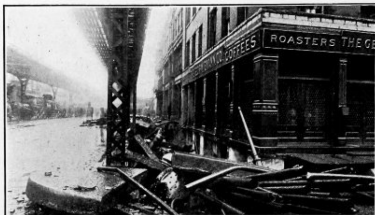
BOILER EXPLOSION, GREENWICH COLD STORAGE CO., NEW YORK, N. Y. TUBES IMPROPERLY ROLLED IN TUBE SHEET
