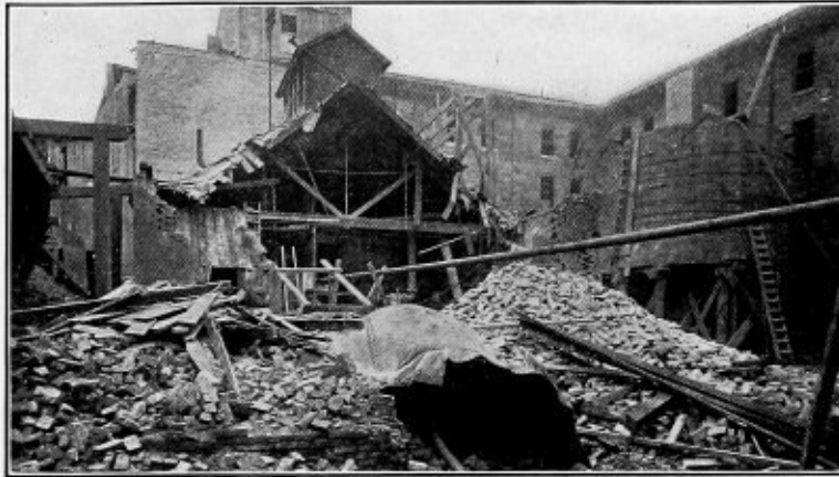
BOILER EXPLOSION, ROBINSON CLAY PRODUCTS CO., MIDVALE, OHIO. 2 KILLED; PROPERTY LOSS, $24,000. BOILER CONNECTED TO BATTERY WHEN PRESSURE WAS DIFFERENT
