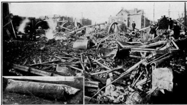
WATER-TUBE BOILER EXPLOSION, ST. LOUIS TRANSIT CO. 7 KILLED; 19 INJURED; PROPERTY LOSS, $112,000. CAUSE, BREAKAGE OF STEAM HEADER
