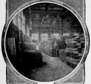
Boiler Lugs and Hangers
