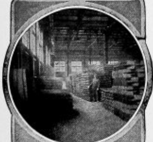
Boiler Lugs and Hangers
