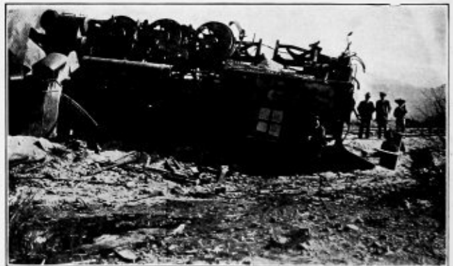
ANOTHER LOW-WATER EXPLOSION
