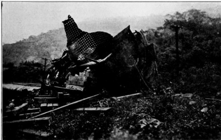
BOILER OF MALLETT COMPOUND ENGINE WHICH EXPLODED FROM LOW WATER
