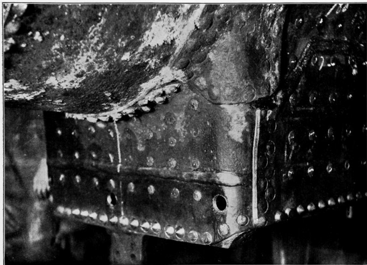
FIG. 4.—THROAT SHEET REPAIRED BY ELECTRIC WELDING
