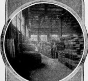
Boiler Lugs and Hangers
