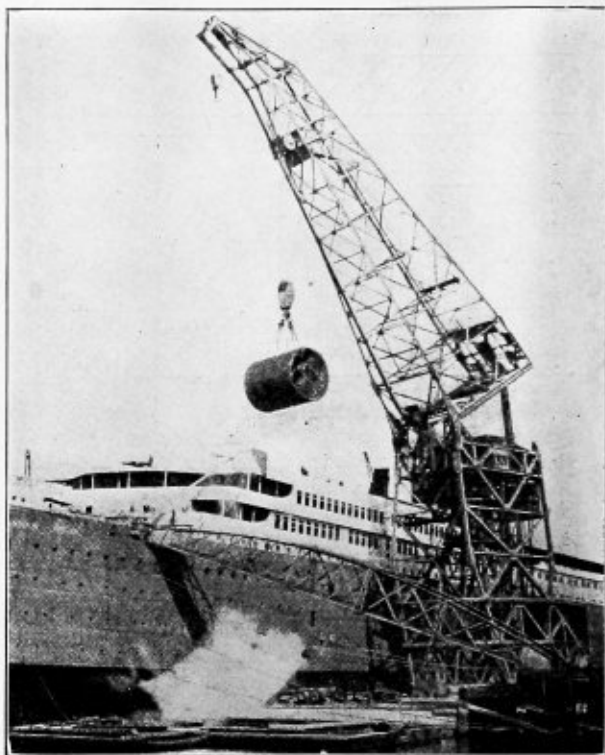
Fig. 2.—Placing Double-Ended Boiler on Board the Britannic
