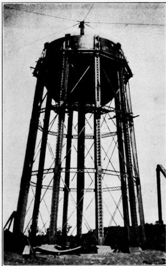
Fig. 2.—Tower Supporting Tank
