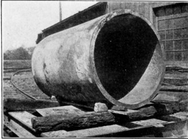
Fig. 1.—2½-Inch Plate, Welded Solid
