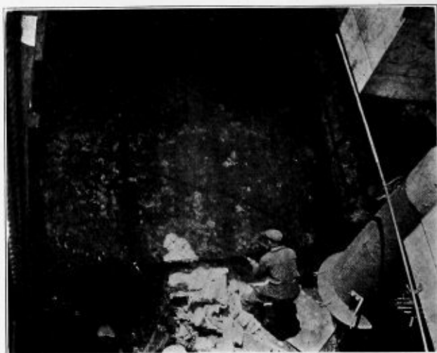
Fig. 3.—Torch Operators Finishing Cut Across Boiler Head
