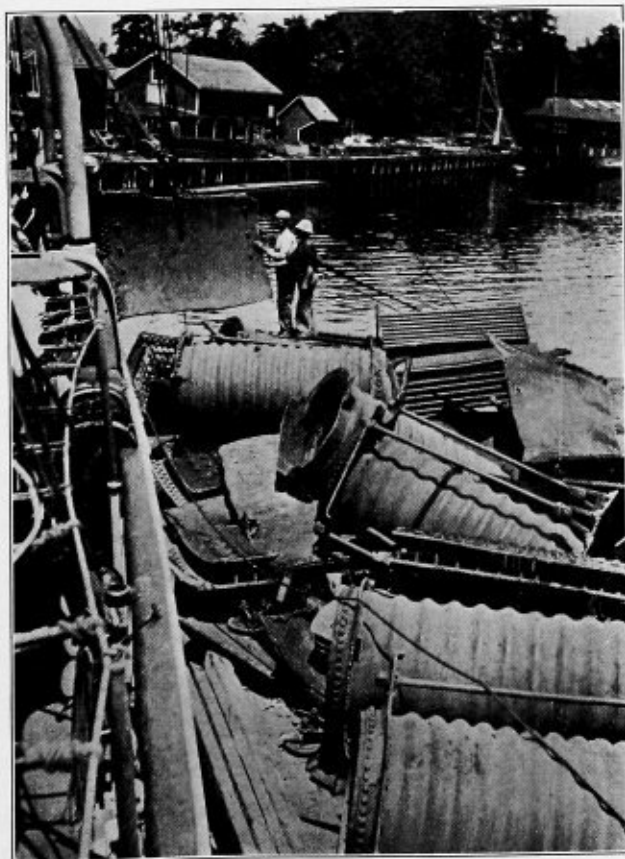
Fig. 5.—Lowering Sections to Scow
