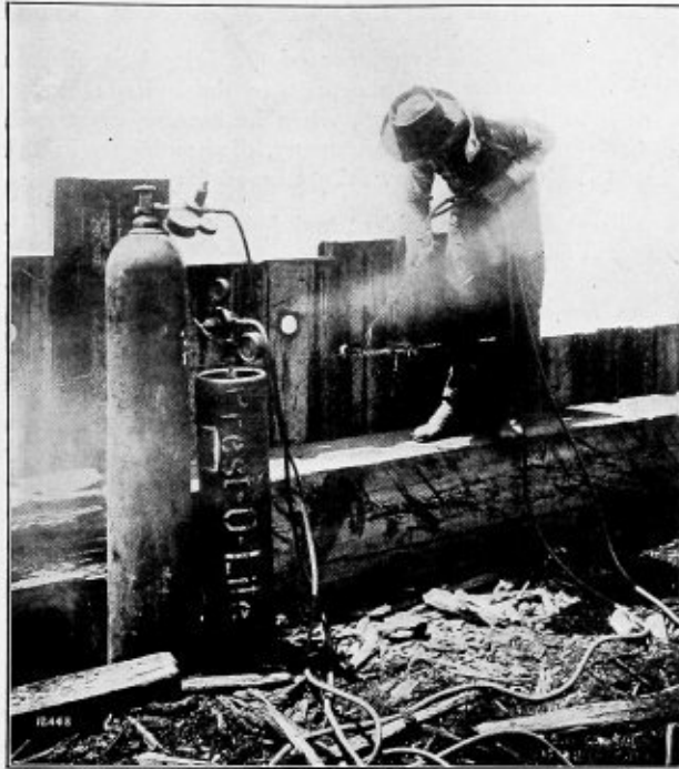
Operator Cutting Sheet Steel Piling with Prest-O-Lite Outfit
