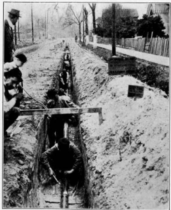
Joining the Sections in the Trench
