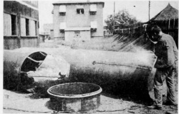
Fig. 5.—Cutting Scrap with Graphite Electrode
