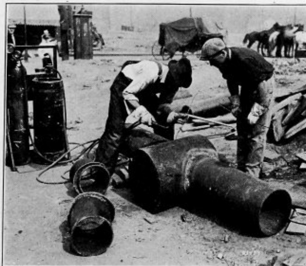
Fig. 4.—Emergency Welding and Cutting Job
