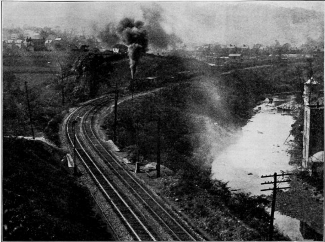
Fig. 3.—Poorly-Fired Freight Locomotive, Emitting Dense, Black Smoke
