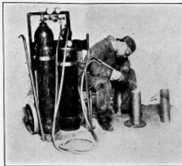
Fig. 1.—Prest-O-Lite Portable Welder
