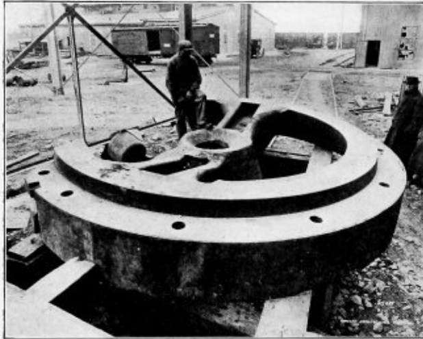
Fig. 5.—Broken Casting Subsequently Reclaimed by Oxy-Acetylene Welding
