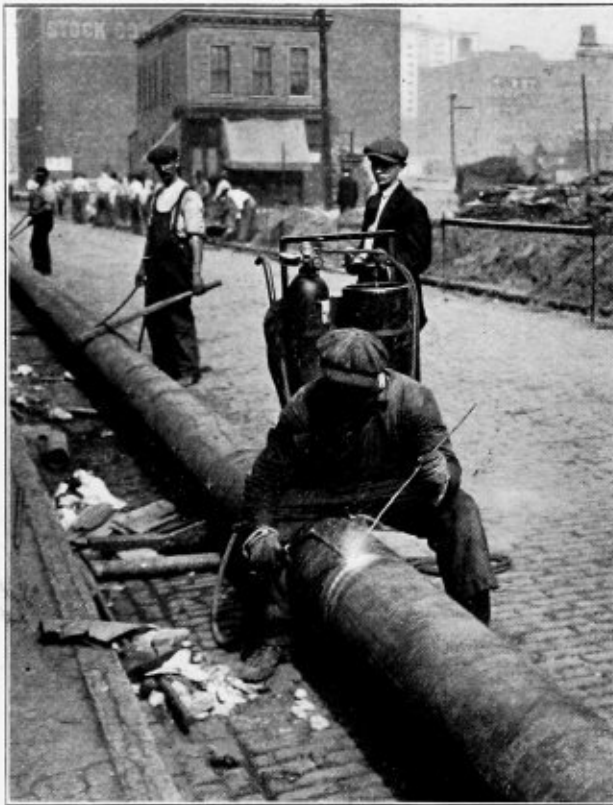
Fig. 1.—Welding Gas Main with Oxy-Acetylene Torch
