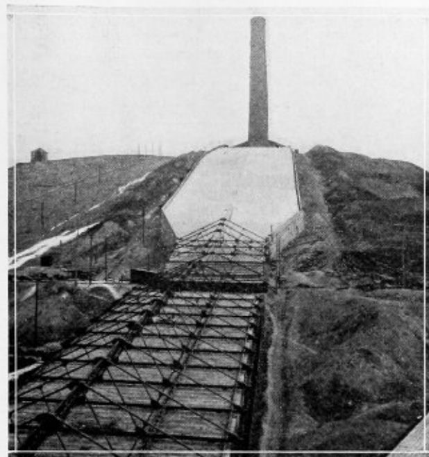
Fig. 1.—Welded Metal Roofed Flue, 120 Feet Wide, 850 Feet Long
