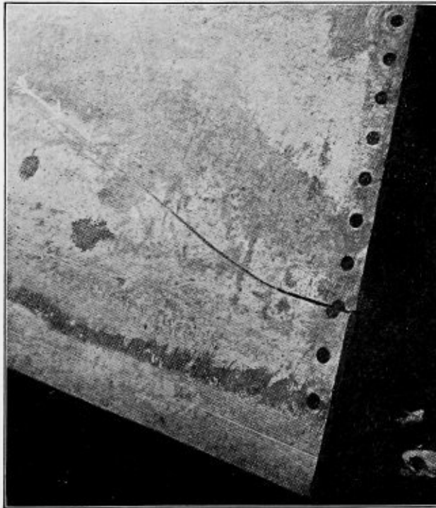
Fig. 1.—Cracked 1-Inch Plate
