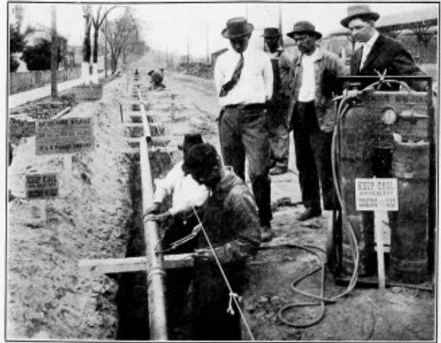
Welding Sections of the Pipe
