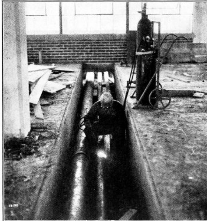
Fig. 5.—The Welding Operation
