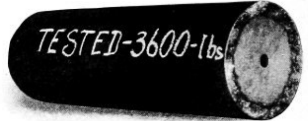
Fig. 4.—High-Pressure Cylinder Welded with Metallic Electrode
