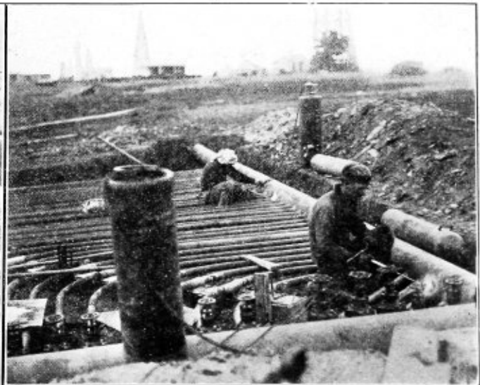
Fig. 3.—Welding in Small Gas-Cooling Pipes
