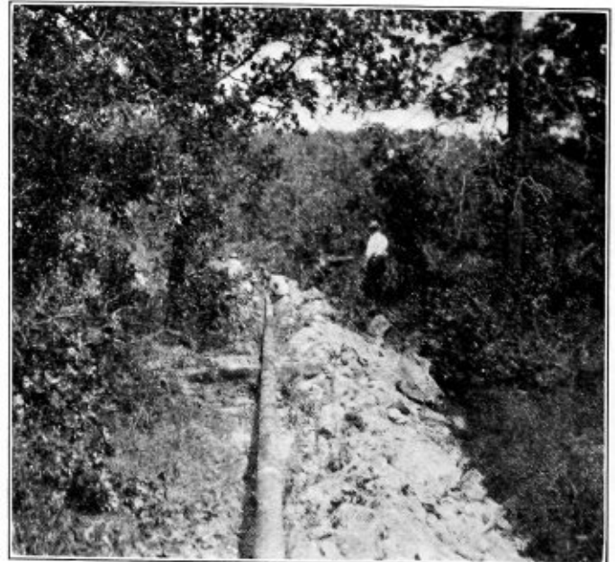
Fig. 6.—Rugged Country Where Pipe was Welded
