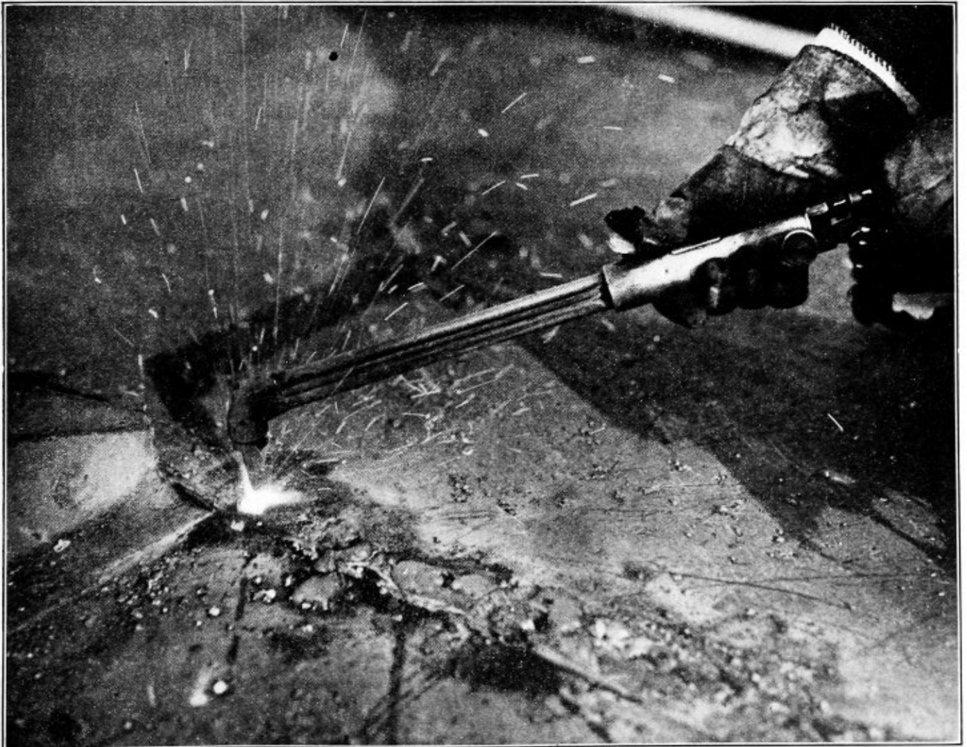
Fig. 1.—Burning or Cutting Off Rivet Heads with Prest-O-Lite Torch
