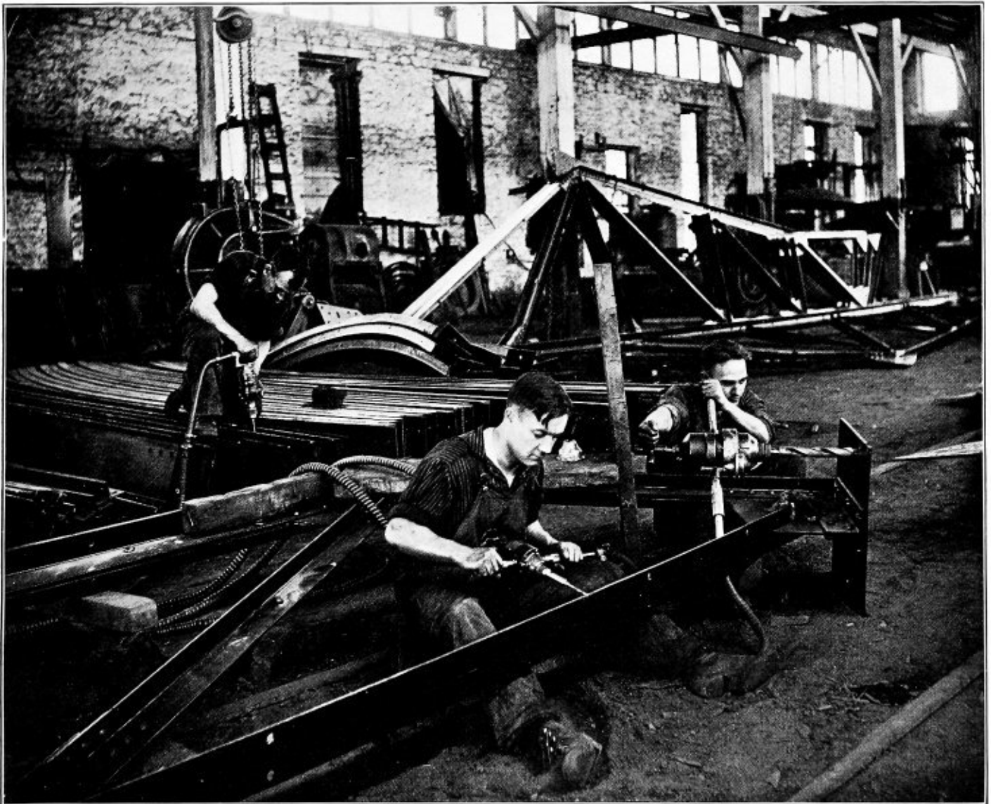
Fig. 1.—Portable Pneumatic Drills at Work in Fabrication of Structural Work
