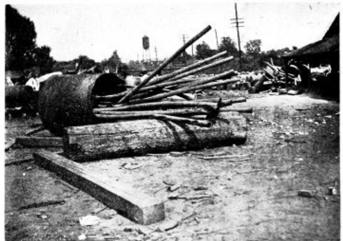
Fig. 3.—Front Portion of Large Boiler
