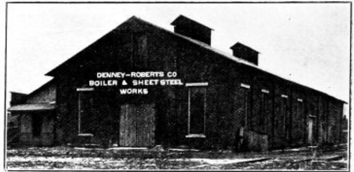
Fig. 1.—Exterior of Denney-Roberts Boiler Shop
