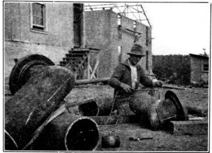
Fig. 1.—Constructing Elbows with Cutting and Welding Torch
