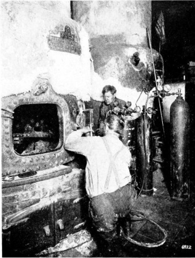
Fig. 2.—Burning Out Staybolts with Oxy-Acetylene Torch
