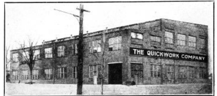
Detroit Office and Salesroom and St. Mary's Plant of Quickwork Company
