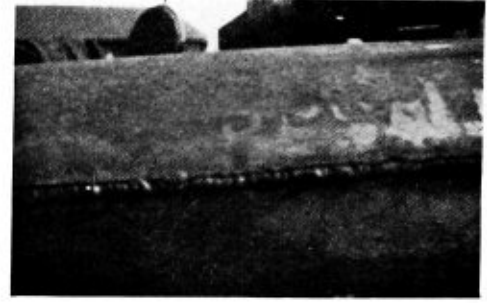
Fig. 7.—Tank No. 2. Part of Bursted Seam Shown in Larger Scale
