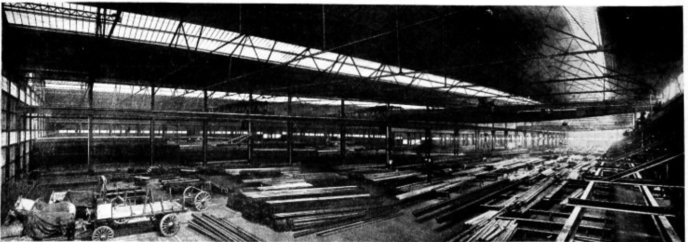
Fig 2.—Interior of Ryerson Structural Warehouse, Chicago
