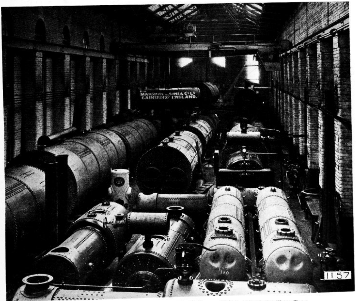
Fig. 11.—Another Interior View Showing the Varied Types of Work Handled in These Shops
