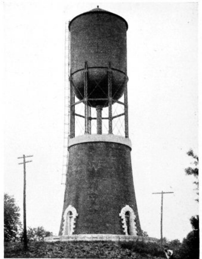
Steel Water Tank, 27 Feet Diameter, 150,000 Gallons Capacity, Built on Brick Tower
