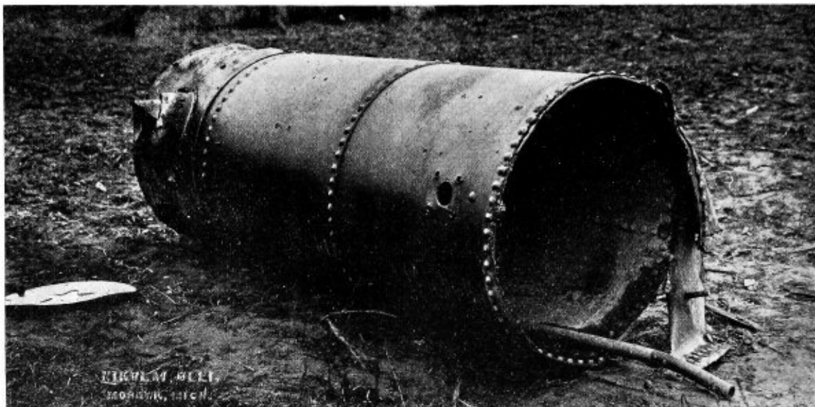
Shell of Exploded Boiler
