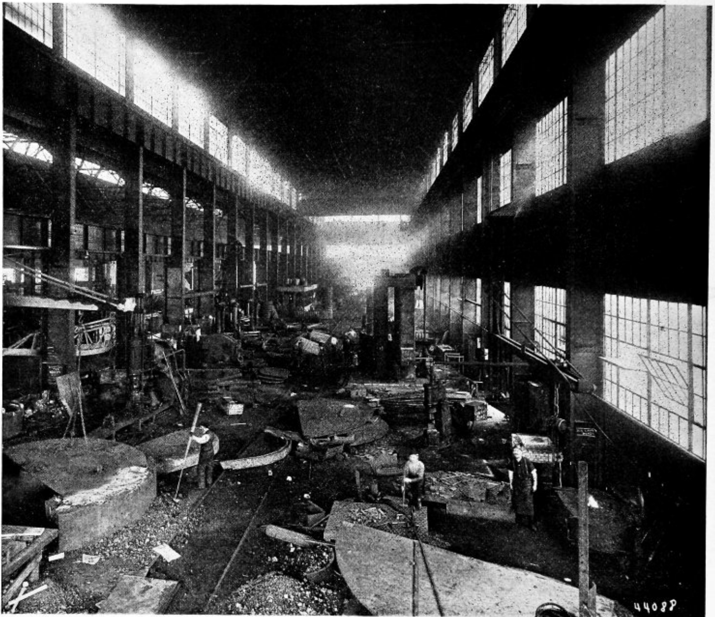
Fig. 2.—Boiler Shop Bay Where Heads Are Shaped
