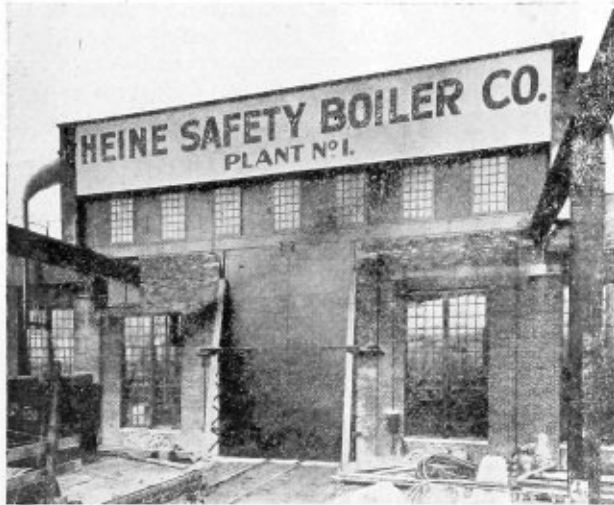
Fig. 1.—Swinging Doors for Special Crane
