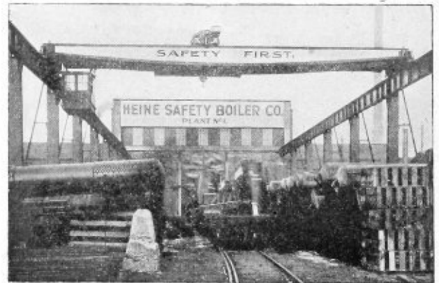
Fig. 3.—Crane Operating in Storage Yard
