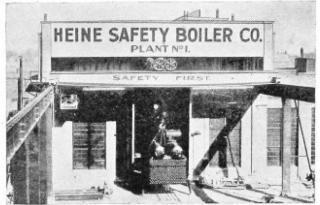
Fig. 2.—Handling Material Through the Doorways
