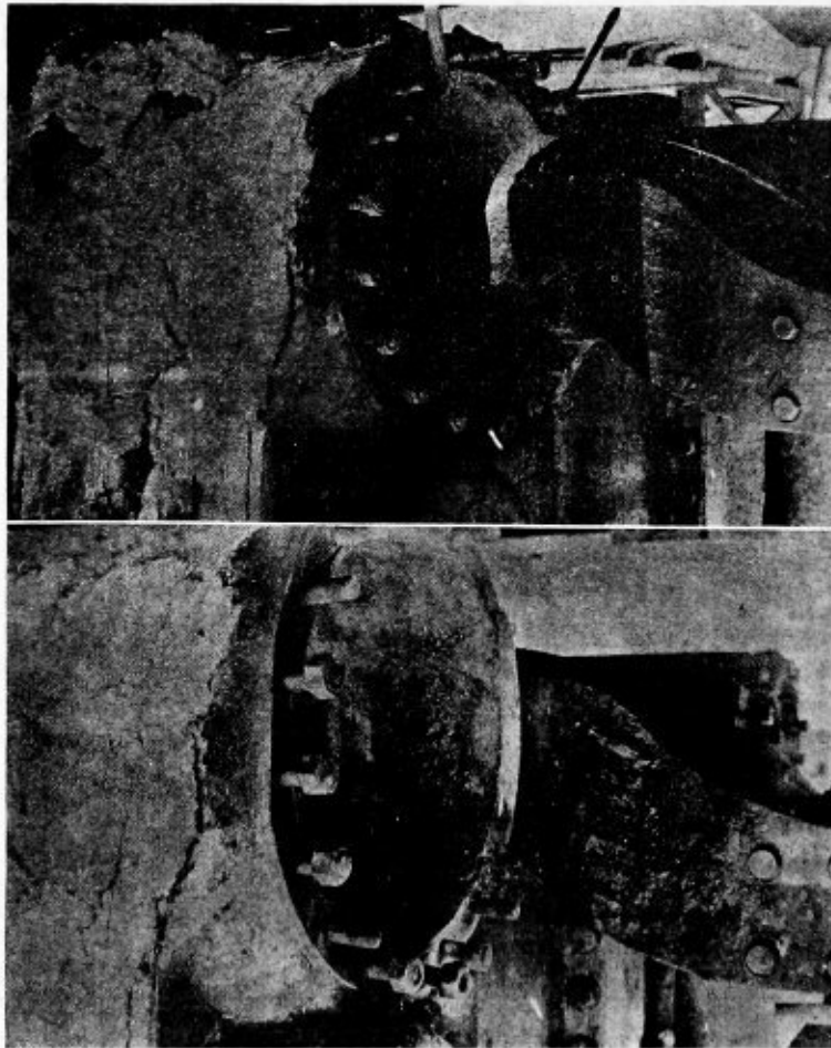
Figs. 7 and 8.—Baldwin Locomotive Cylinder Before and After Welding in Position
