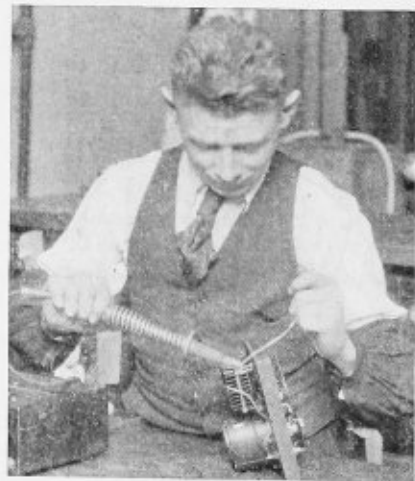
Electric Soldering Iron in Use on Electrical Apparatus
