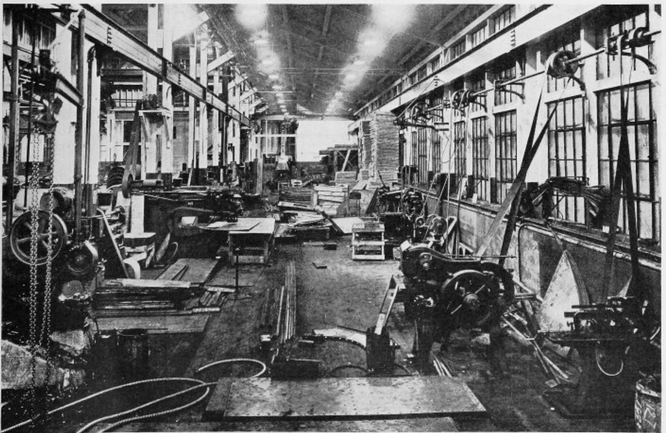
Fig. 12.—East Bay of Shop in Which Department Casings Are Made and Tubes Bent Ready for Installation
