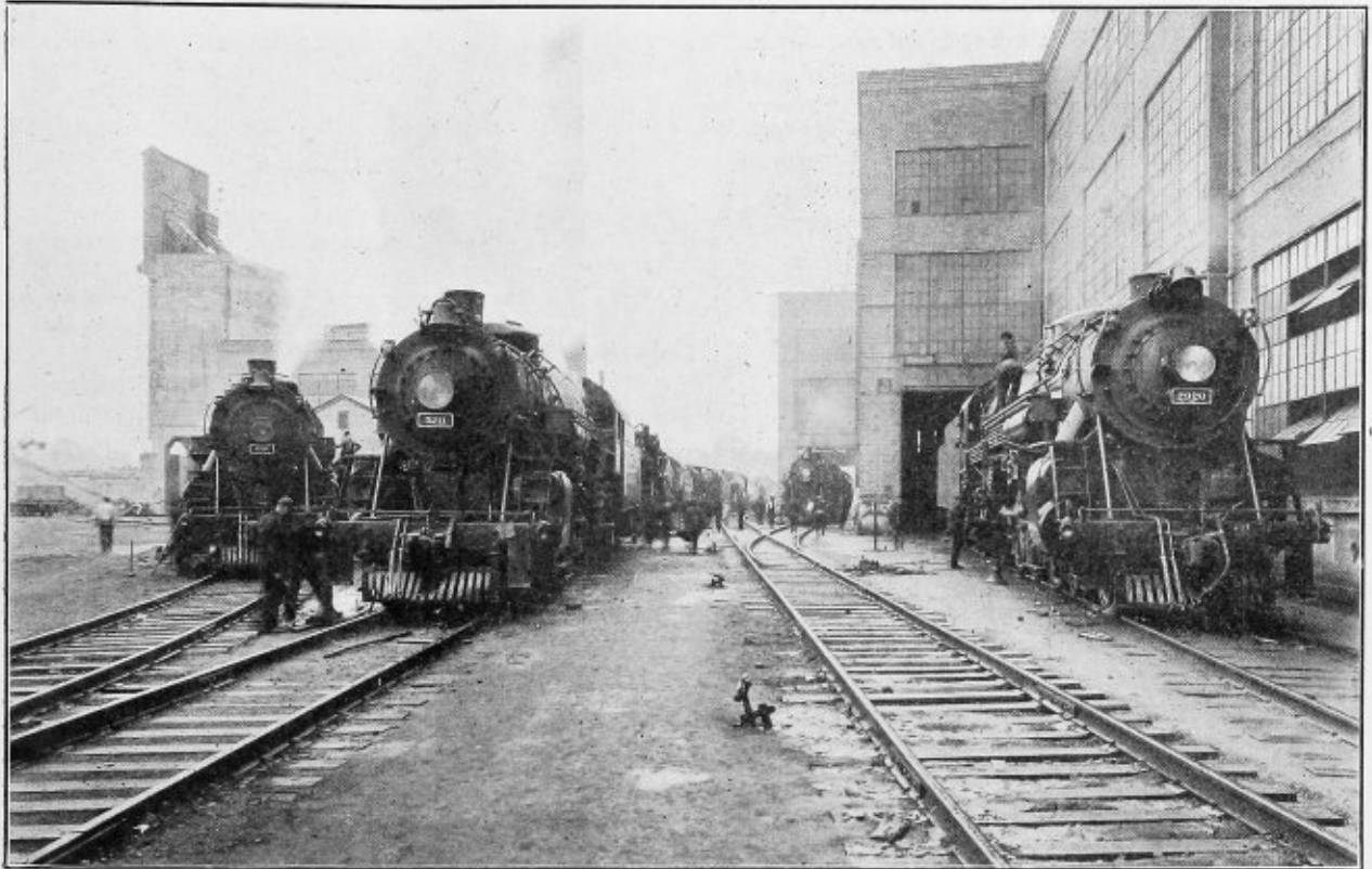
Finishing Tracks at the Eddystone Plant of the Baldwin Locomotive Works
