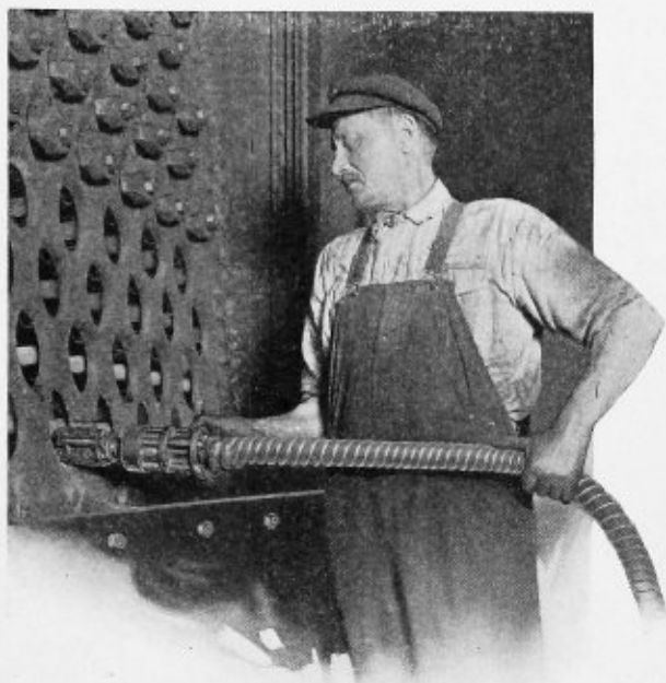
Fig. 1.—Roto Tube Cleaner With the Type A. D. Motor in Use
