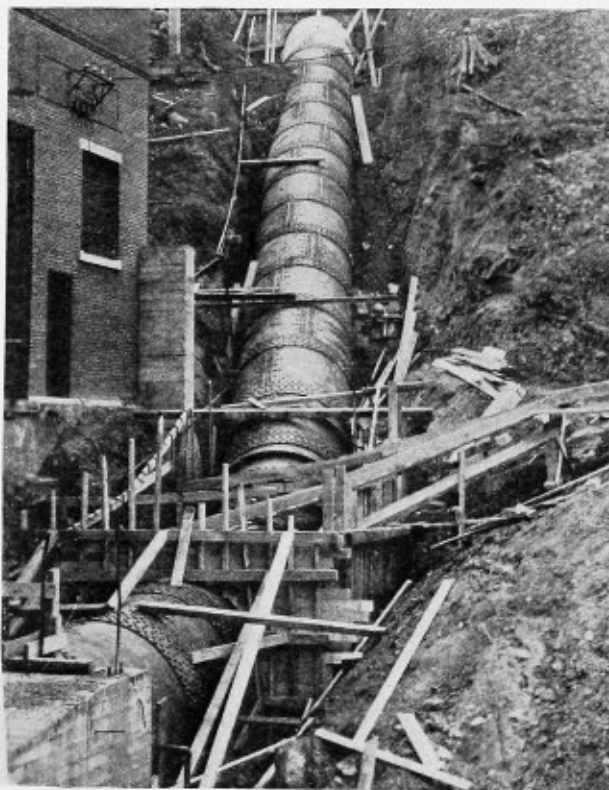
Penstock Installed at Fond du Lac (Minn.) Power Station
