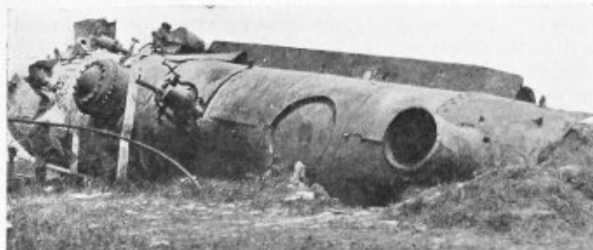
Fig. 4.—Explosion Which Threw Boiler Nearly 400 Feet from Point of Accident
