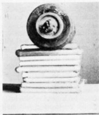
Fig. 8.—Bottom Water Glass Cock Stopped Up Causing Incorrect Water Level Indication
