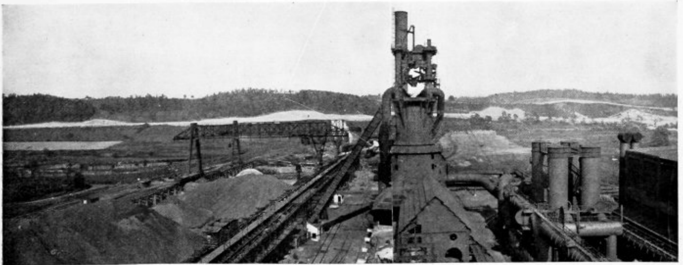
General View of Blast Furnaces and Stock Yard, Showing Method of Handling Materials
