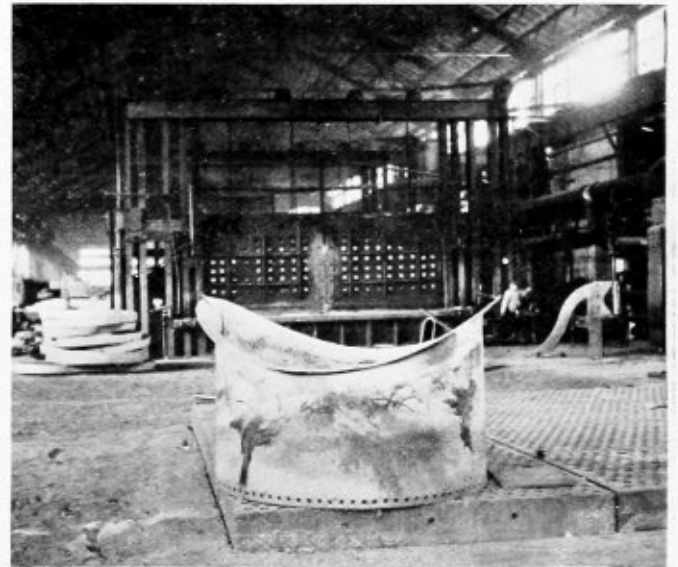
Fig. 3.—Fifty-four Inch Dome Sheet for Tank Car
