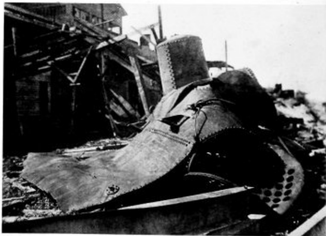
Destruction Caused by Lap Seam Crack Explosion
