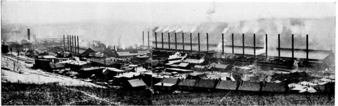
Panorama of Midvale Steel and Ordnance Plant at Coatesville, Pa., Showing the Open Hearth Plant, the Rolling Mills and Settlement of Steel Workers
