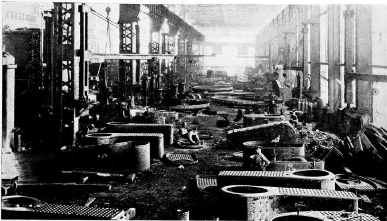
Fig. 1.—Side Bay of Federal Boiler Shop with Combustion Chambers Under Fabrication
