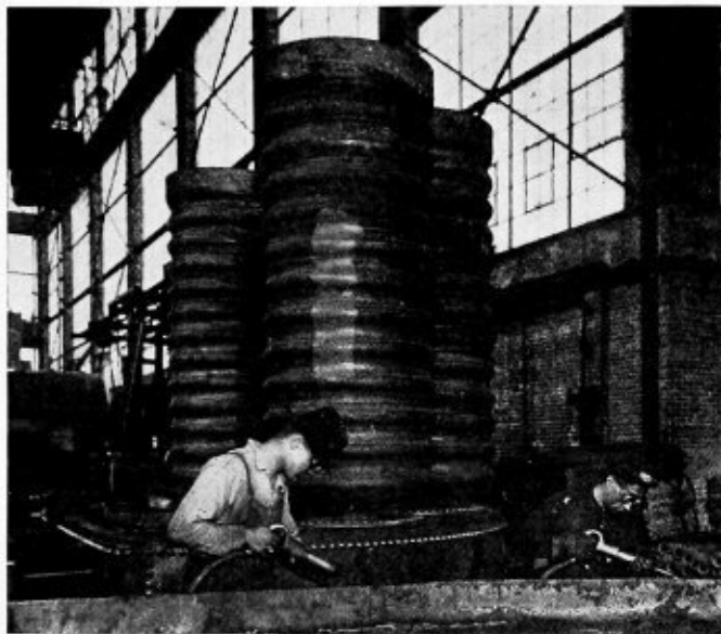
Fig. 11.—Goggles are Necessary Equipment for Such Operations in the Boiler Shop
