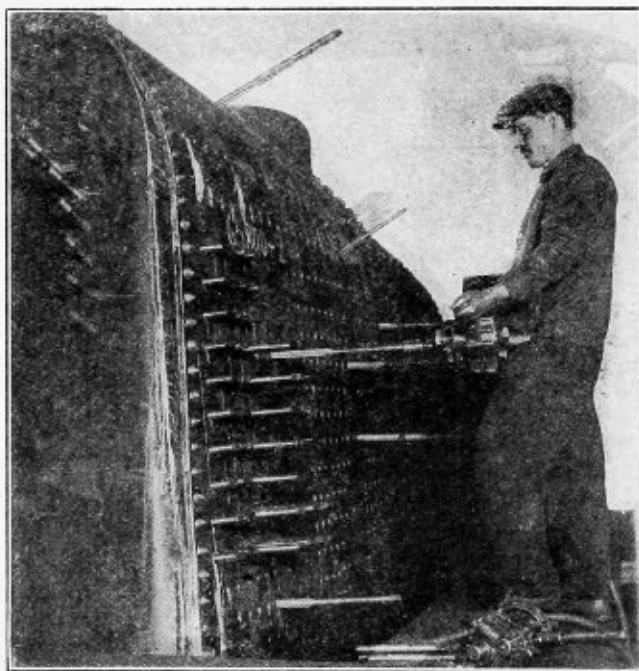
The "Maxitap" in Use on a Locomotive Firebox
