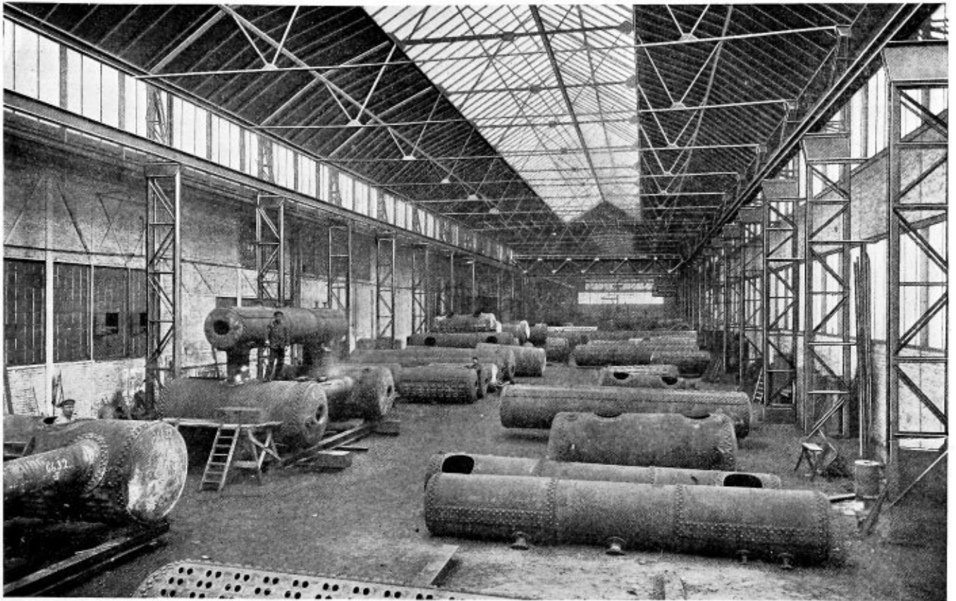
Fig. 3.—Assembling Boilers at the Dürr Shops. Garbe Plate in Foreground
