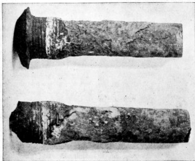
Fig. 2.—Top View Shows Bolt Taken from Sheet After Explosion. Lower—Extent of Corrosion
