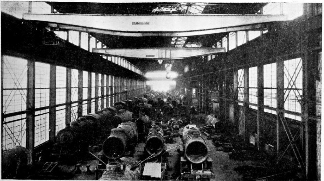
General View of Work in the Erecting Shop
