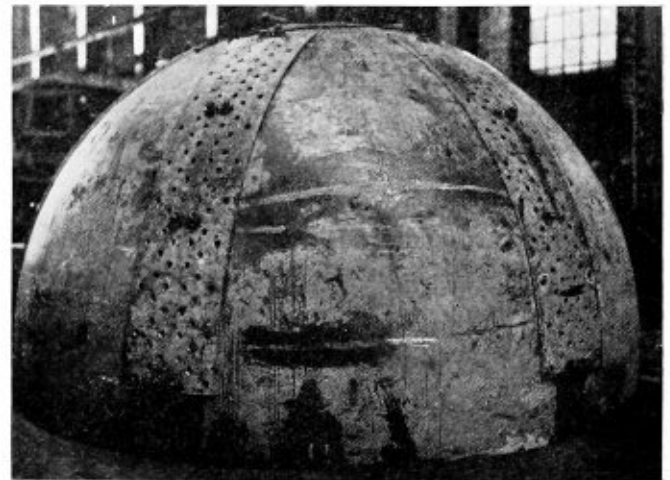
Fig. 3.—Head in Process of Assembly
