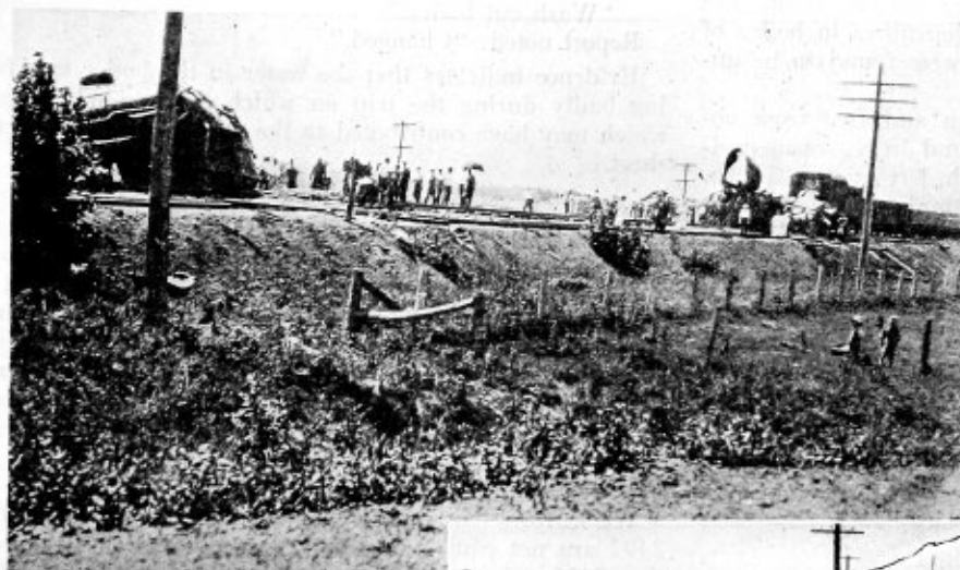
Position of boiler and running gear after explosion
