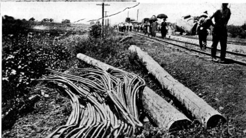
Superheater units were thrown one hundred and fifty feet from boiler
