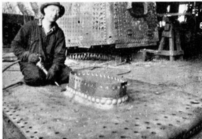
All Fire Doors Are Riveted
