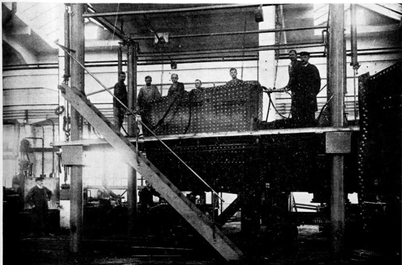
Fig. 8—Time and Labor Saved by Arrangement of Hammers for Riveting Stay Heads
