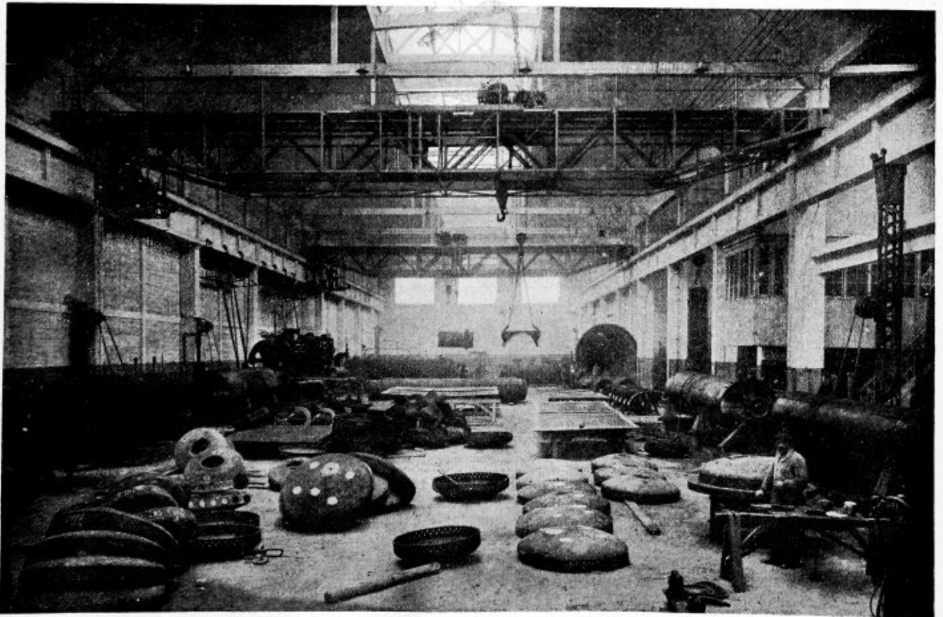
Looking Down the Main Bay of the Boiler Shop
