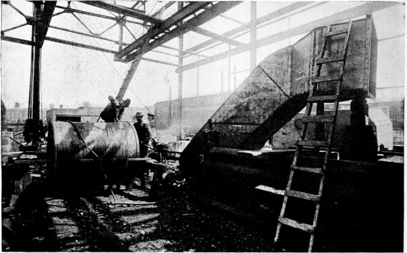
Elbow, chute and tank erected in field
