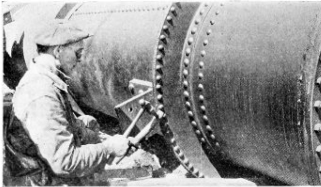
Simple kink eliminates danger from holding-on a chisel
