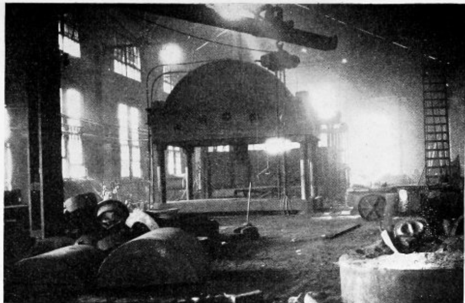
Fig. 18.—550-ton flanging press and furnace
