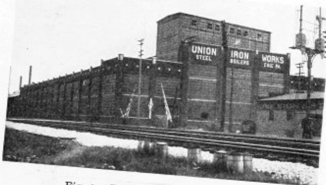
Fig. 1.—Exterior view of boiler shop
