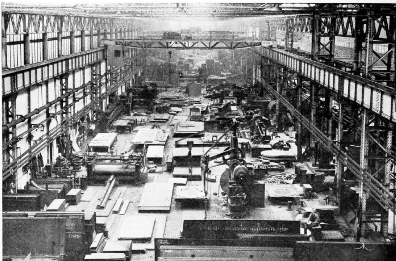
General view of Scotswood boiler shop, north bay, looking east
