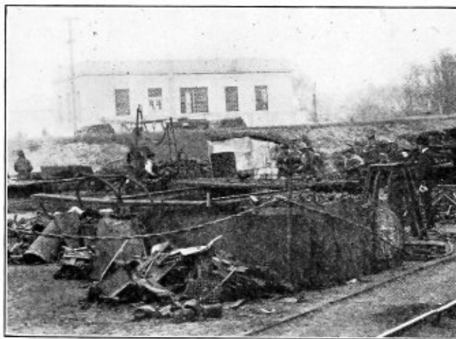
View showing reclamation plant of scrap yard equipped with protective device for acetylene outlet
