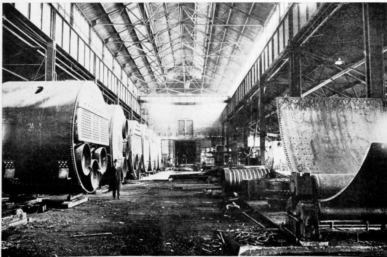
Looking down the center bay from the riveting tower
