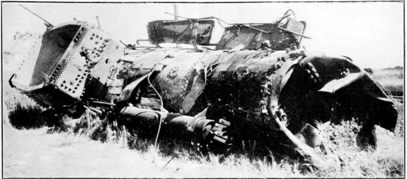
Fig. 1.—Boiler was thrown 305 feet in this low water explosion
