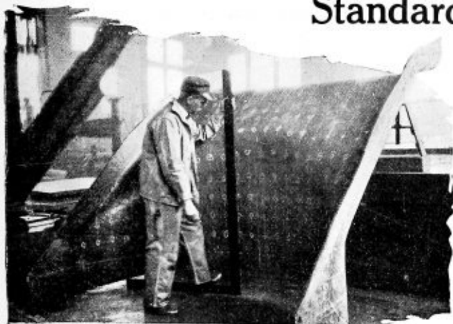
Laying out a throat sheet
