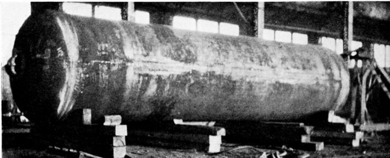
Completed tank built for 300 pounds pressure
