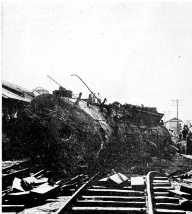
Fig. 3—Result of crown sheet failure on oil burning locomotive
