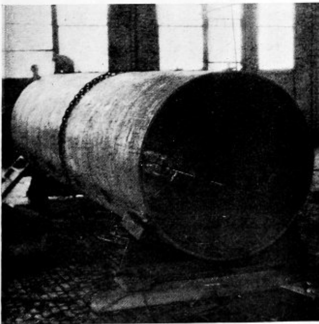
Heavy plate used in tank ready for welding
