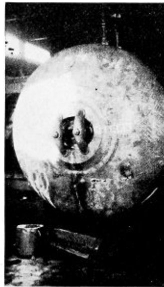
Fig. 19.—End of tank showing new manhole ring
