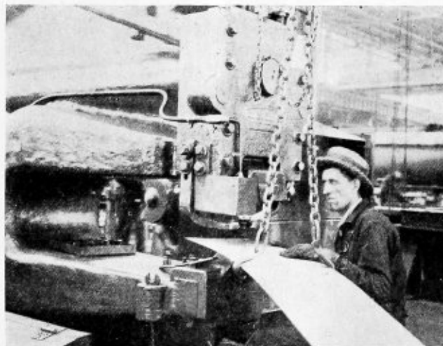
Boiler plate at the punch and shears
