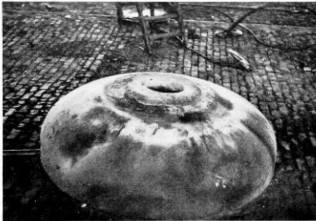
Completed weld on handhole reinforcing ring
