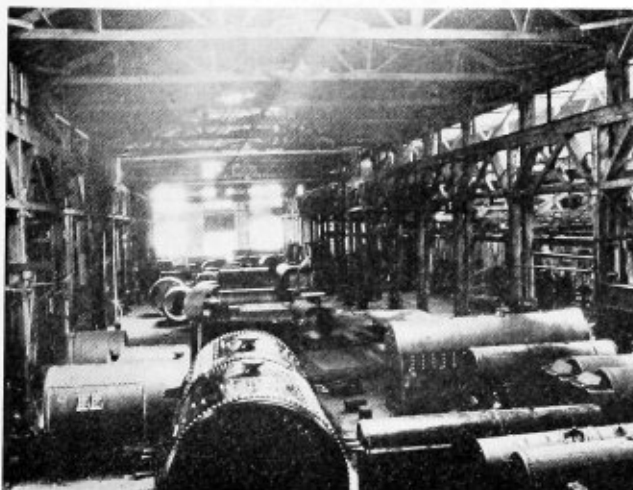
General view of the shop
