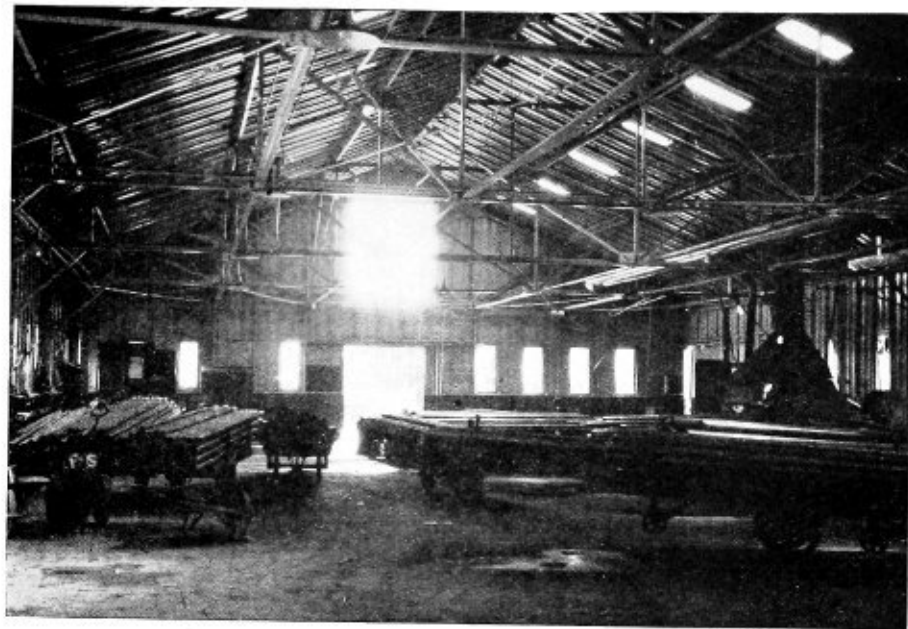
Safe-ended tubes on trucks ready for installation in boilers
