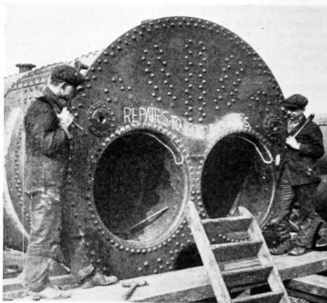
Welding used for repairing a Lancashire Boiler
