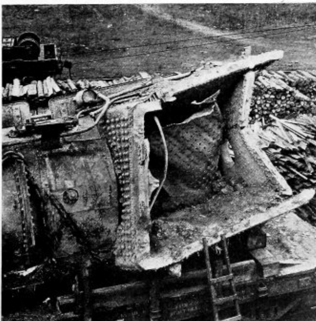
Fig. 3.—Crown sheet failure due to low water caused this accident
