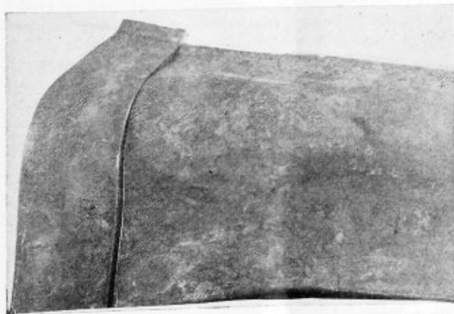
Fig. 2.—View showing details of ruptured area
