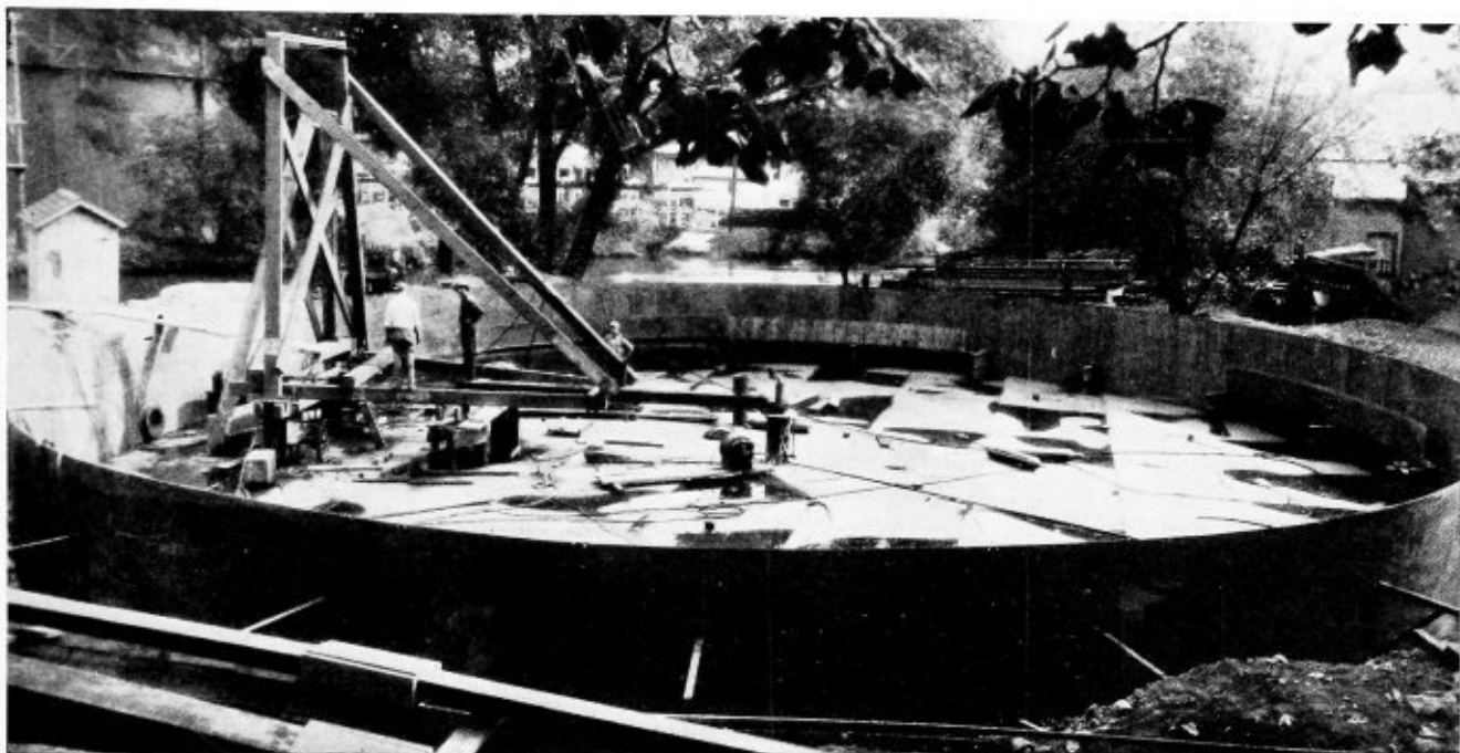
Fig. 1.—Early stages in construction of gas holder
