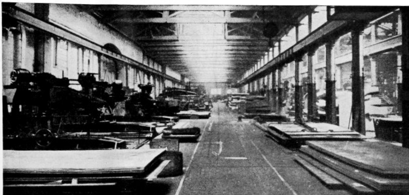
General view of machine bay in boiler shop
