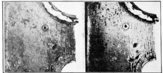
Fig. 2, Left—This view shows the strain lines and pitting of the plate between the staybolt hole and the arch tube hole; Fig. 3, Right—The same as Fig. 2, but polished to intensify the lines
