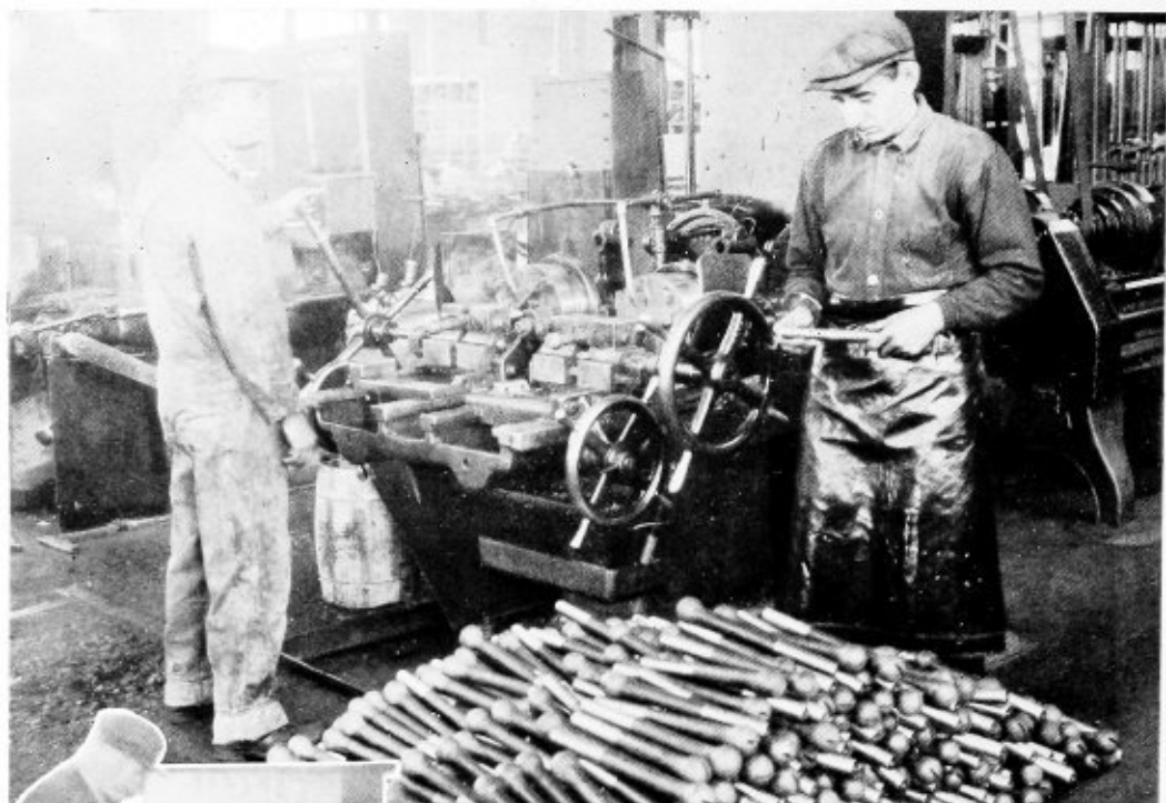
(Above)—Machine set up for threading flexible staybolts
