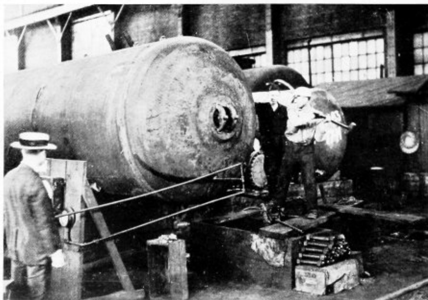
Fig. 2.—Pressure-impact test of pressure vessel
