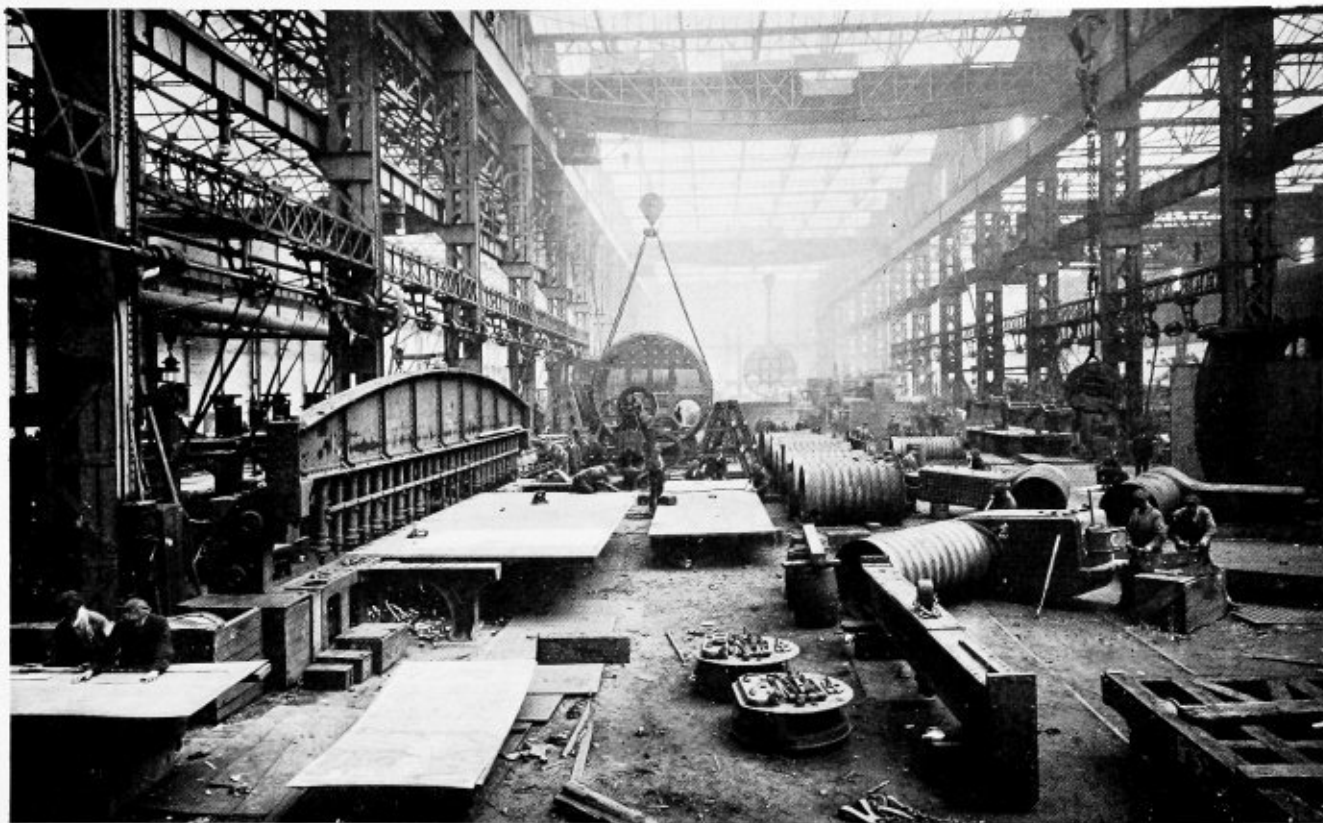
General view of the boiler shop at Birkenhead
