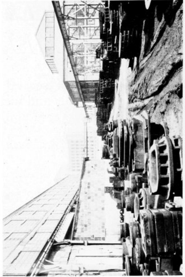
General view of the upper bay showing an R. D. Wood flanging press and its furnace
