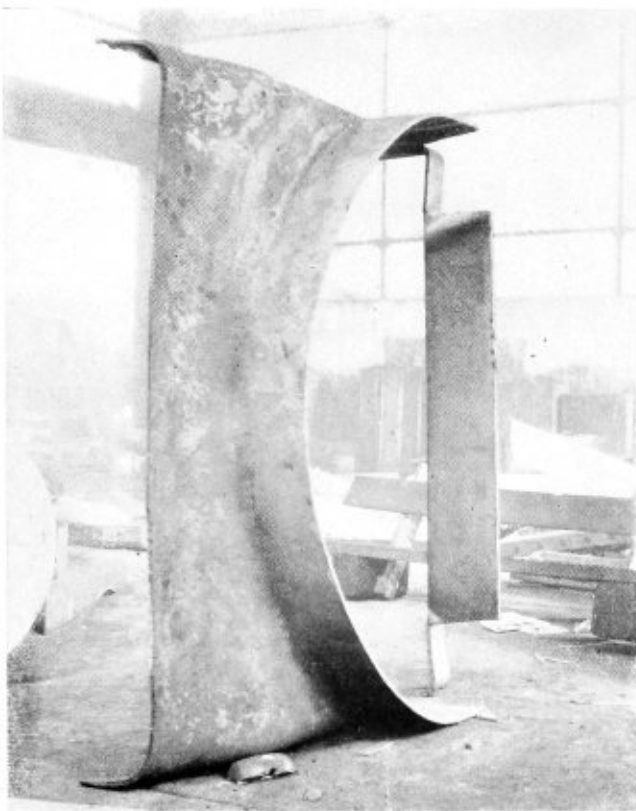
Fig. 51.—Throat sheet after coming from press with tie piece still in place
