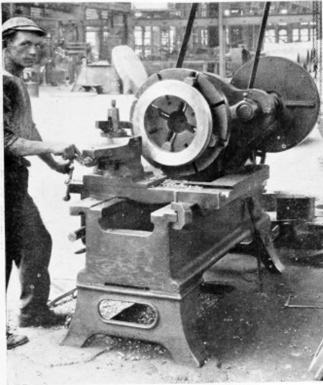
Steam pipe ring set up in a lathe for machining
