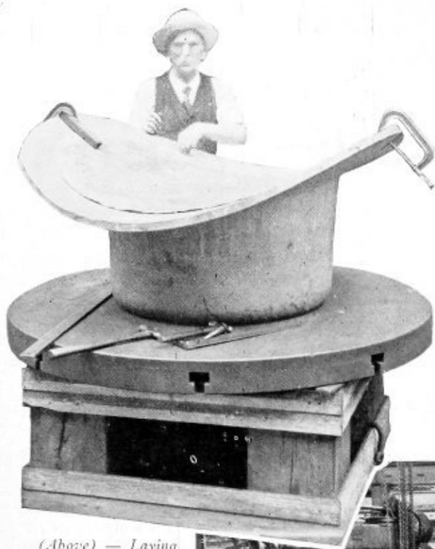
(Above) — Laying out the dome flange holes and edge
