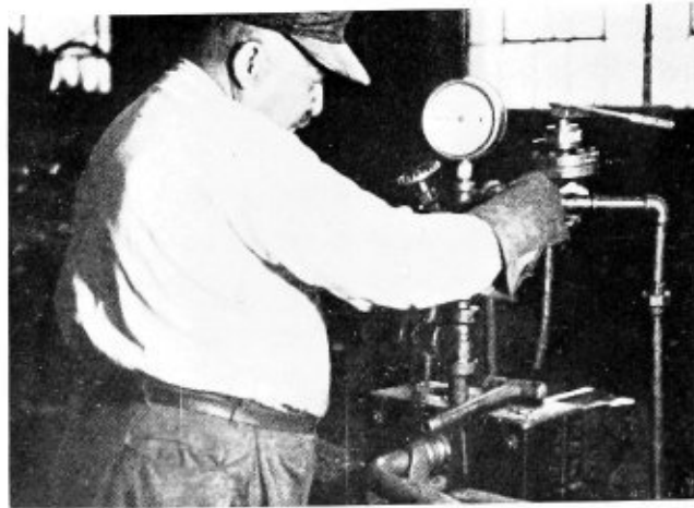
Every unit is given a 1000-pound hydrostatic test
