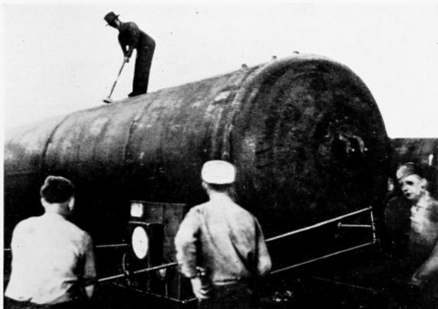
Fig. 4.—Impact test for longitudinal seam of pressure vessel
