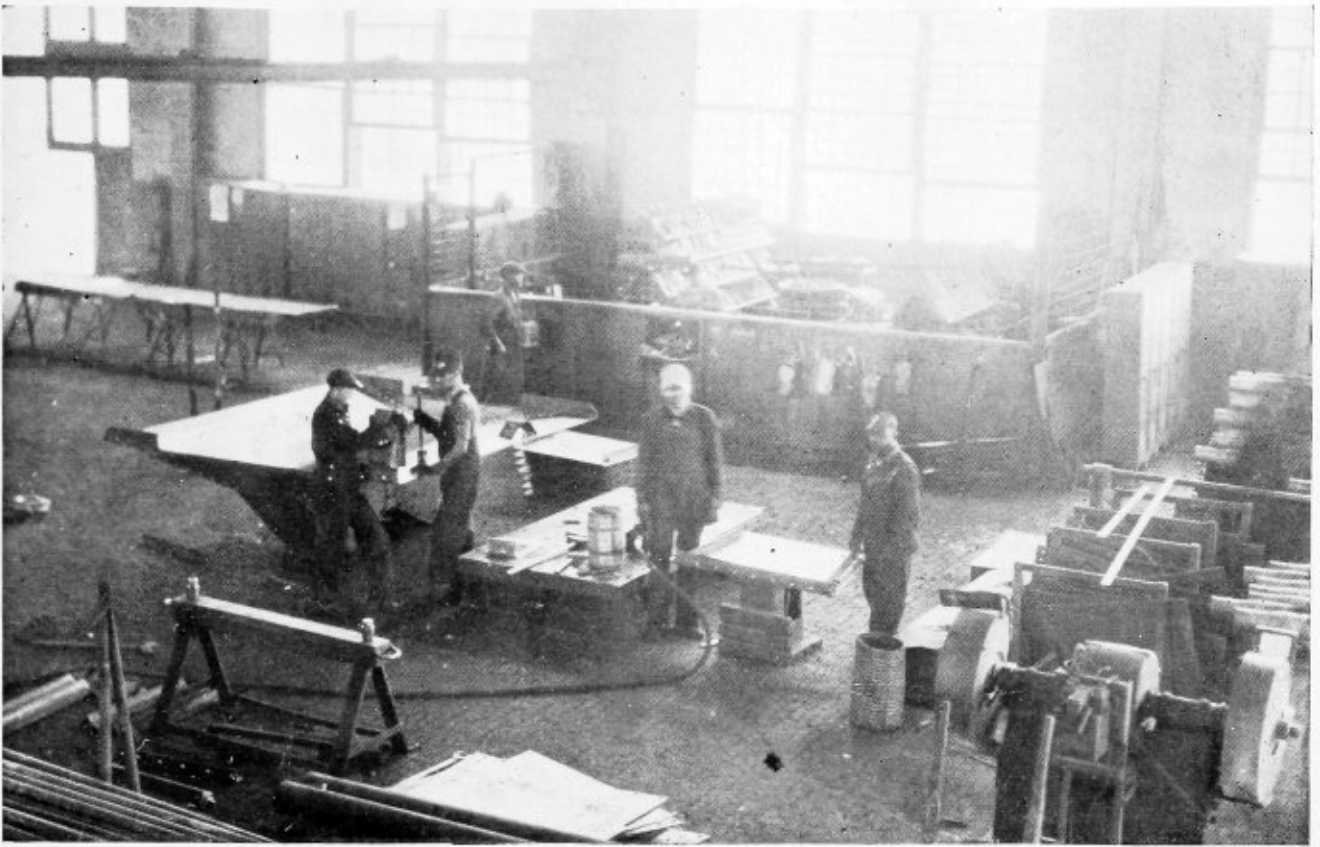
Ashpan shop and tool room
