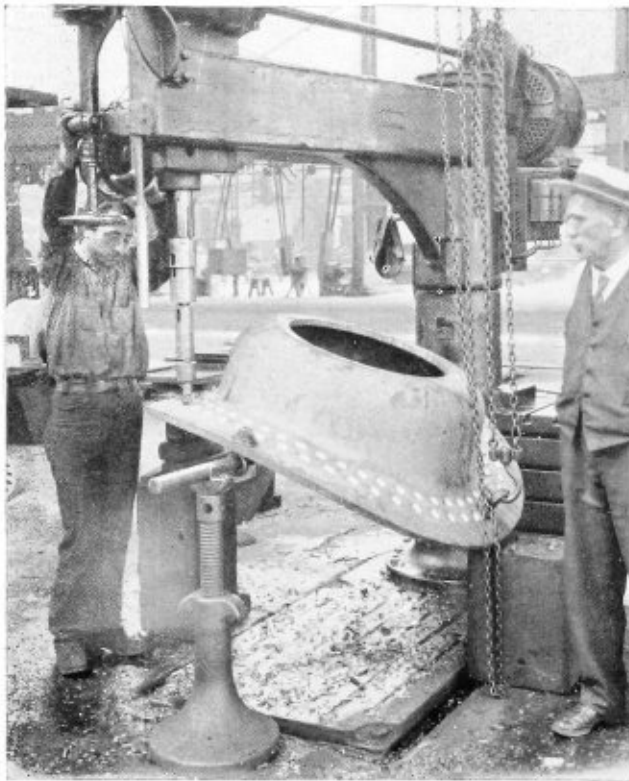
Countersinking the dome flange rivet holes
