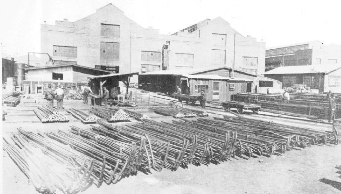
Re-manufacturing unserviceable superheater units
