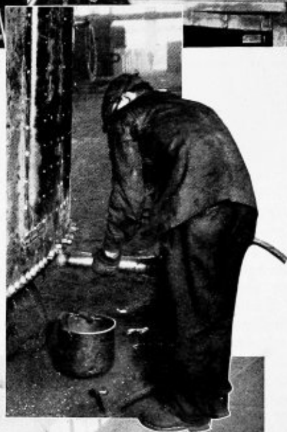
Hand fitting odd firebox rivets
