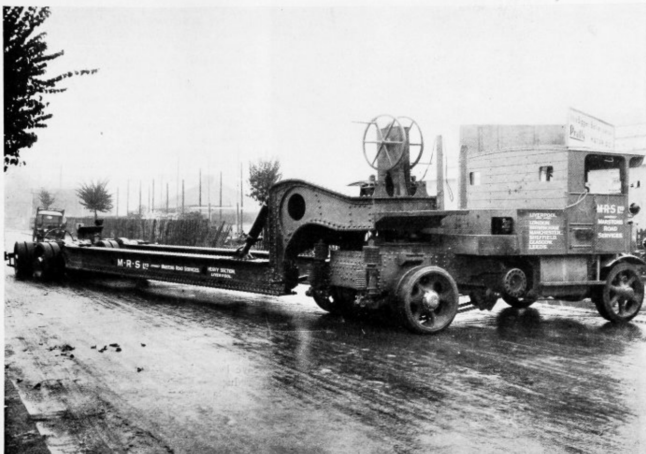
Fourteen wheel truck and trailer used for hauling boilers
