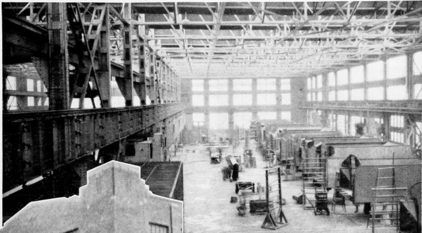
A well-equipped section of the boiler shop is devoted to the handling of tank maintenance
