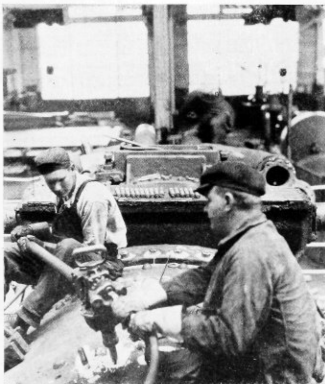
Boiler tapping operation
