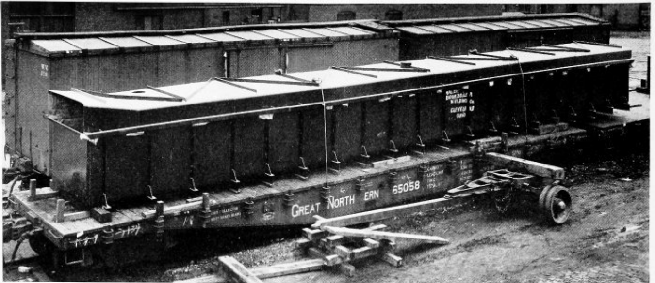
Lead-lined welded steel pickling tank loaded for shipment
