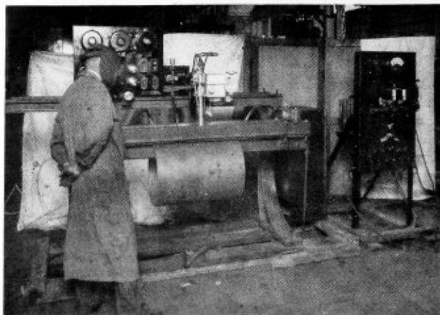
The General Electric automatic welding machine for use with the atomic-hydrogen welding process
