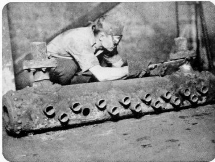
Fig. 1.—Grates and header easily removed with cutting torch
