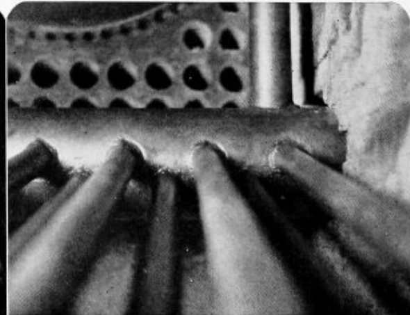
Fig. 3.—Tubes properly spaced and welded to header
