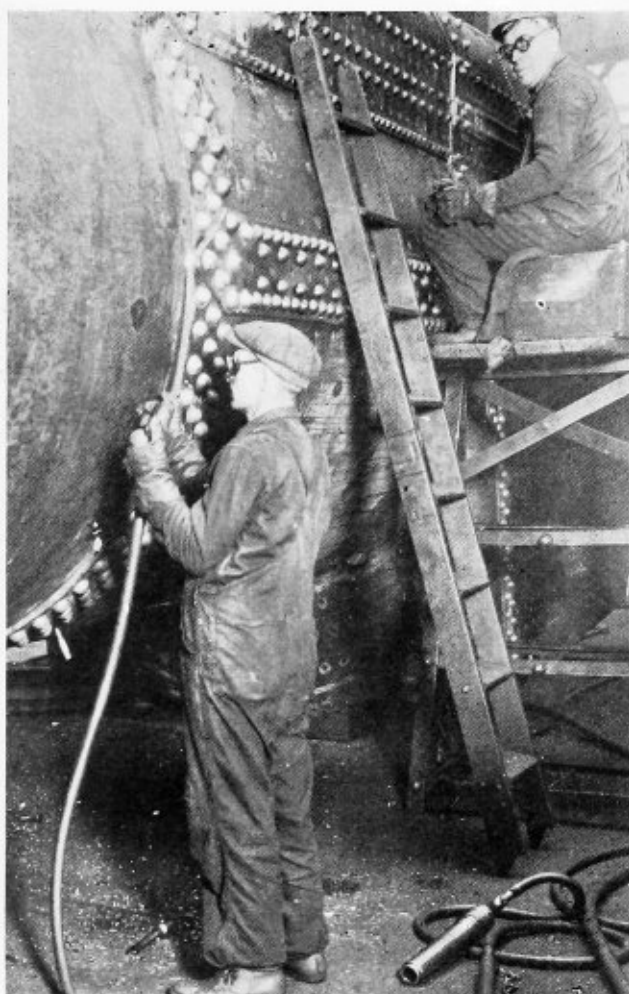
Calking boiler seams
