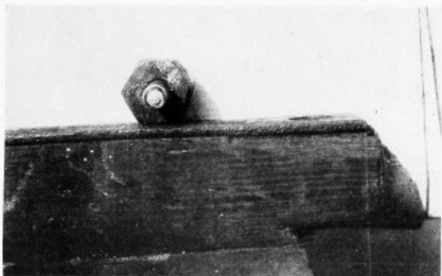
Fig. 7.—Bottom nipple of water glass closed with mud
