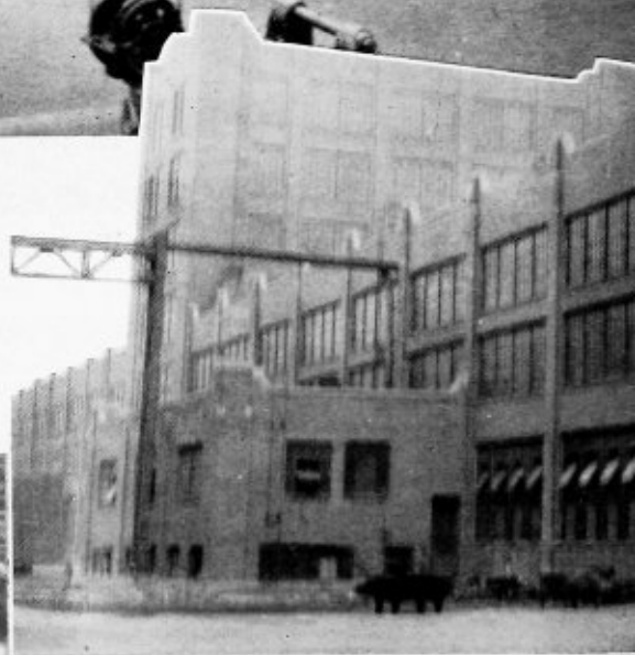
The Illinois Central Paducah boiler shop (right) is one of the best arranged and equipped in the country
