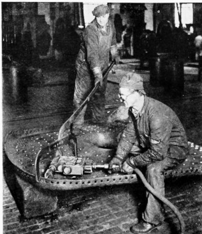
A special lever arrangement facilitates the rapid counter-sinking of rivet holes in a firebox door-sheet flange
