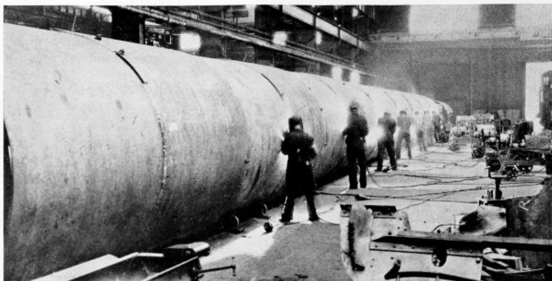
Fig. 1.—C. B. & Q. welded tie-treating retort
