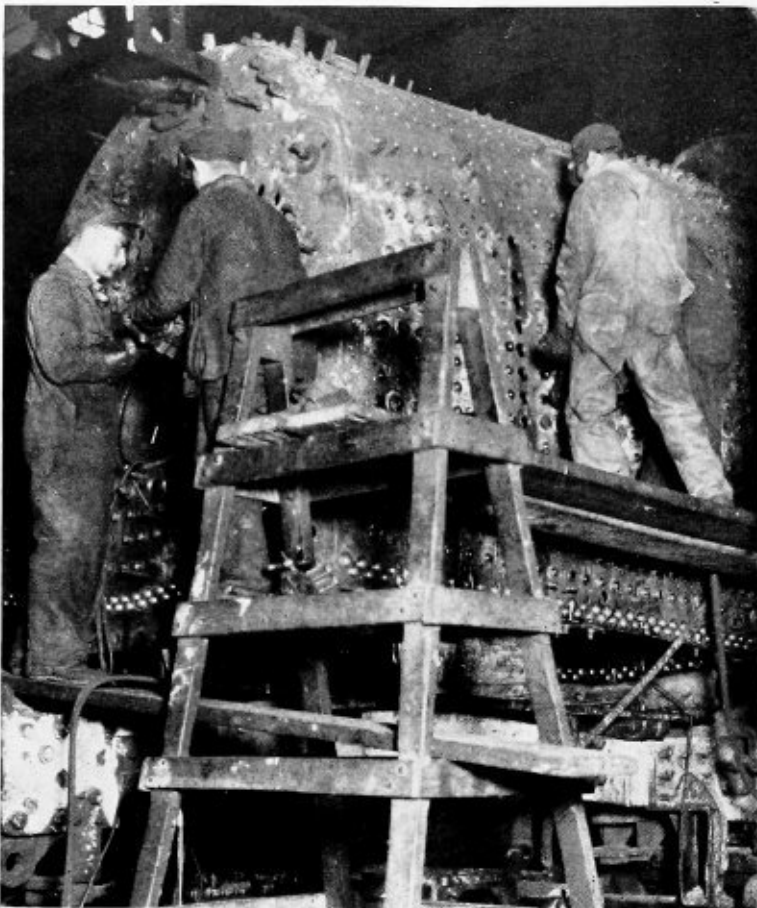
Fig. 8.—Operations incidental to fitting up the back end assembly at one of the Erie shops
