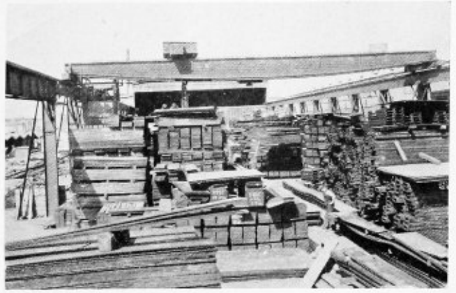
Unprotected plate and shape storage
