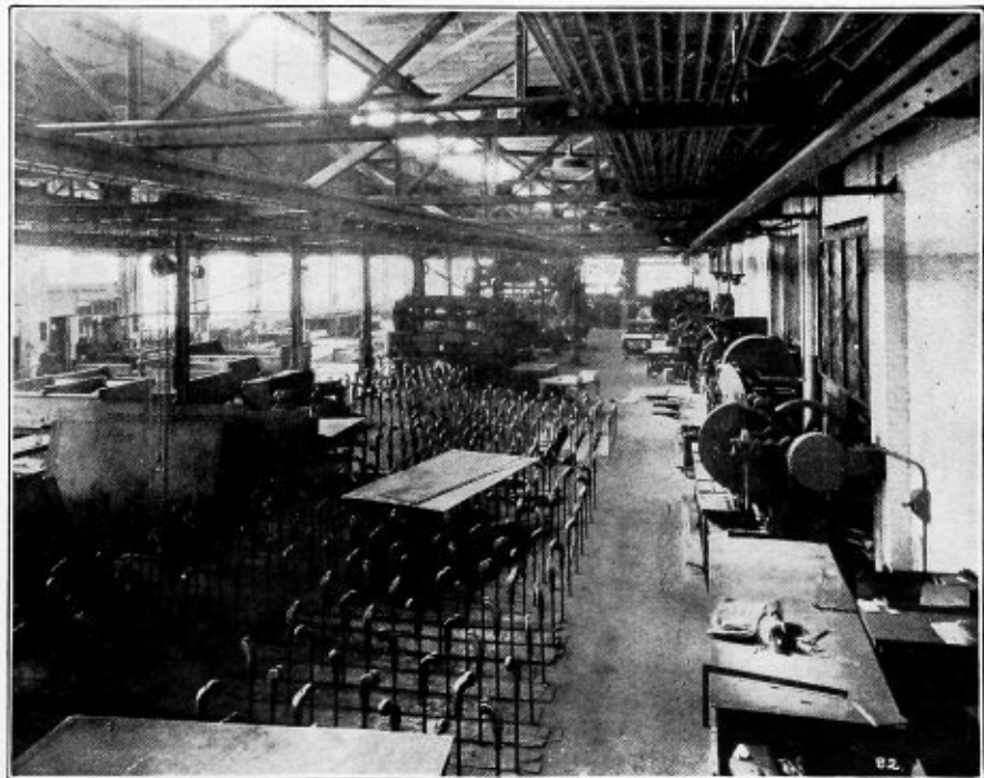
Sheet metal marking, shearing and punching department with pipe stand rollers for ease in sheet handling
