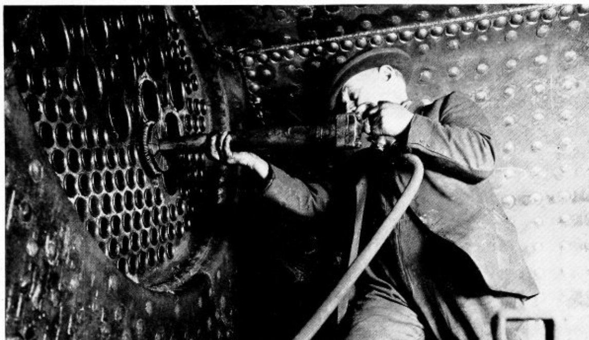
Fig. 1.—Prossering superheater tubes in a locomotive boiler
