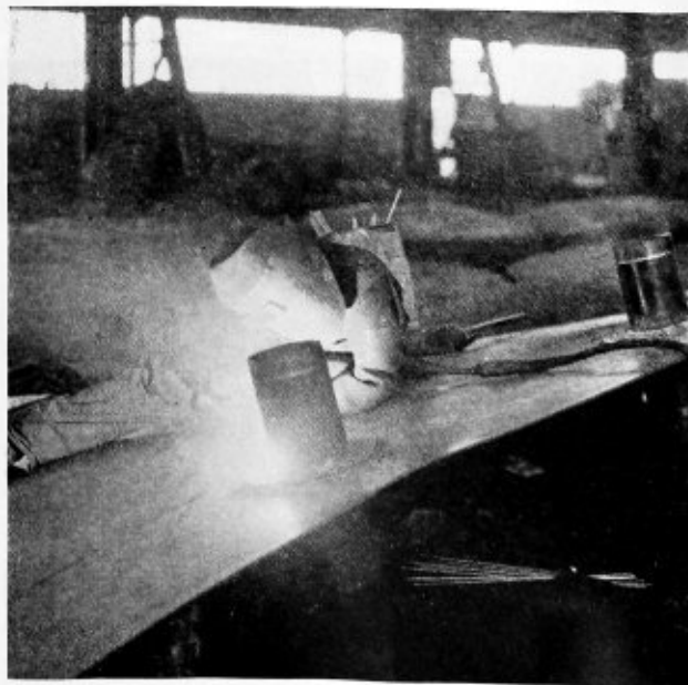
Fig. 2.—Welding plates for erection
