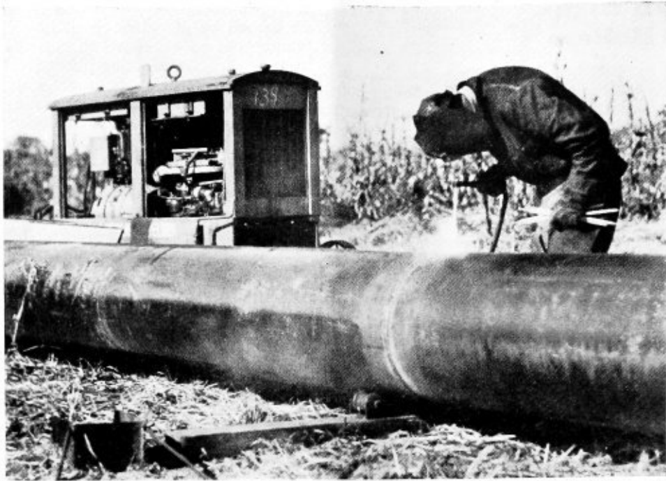
Fig. 1.—Arc welding field connections on pipe line
