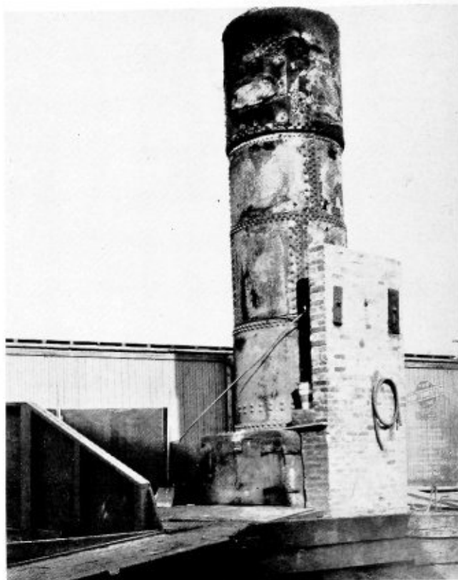
Scrap locomotive boiler used as an incinerator
