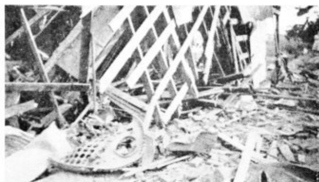
Above—Middle and rear courses of Neal, Georgia, boiler Below—Where eight were killed in cotton gin boiler explosion
