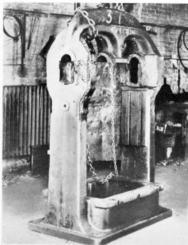
Cast-iron punch press frame repaired by arc welding
