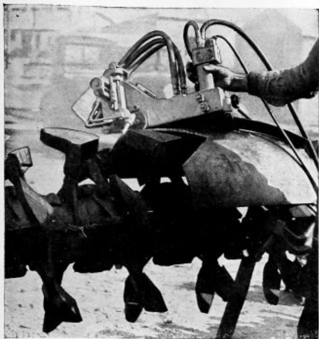
Removal of surplus steel
