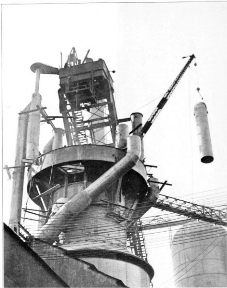
Blast furnace uptakes under erection
