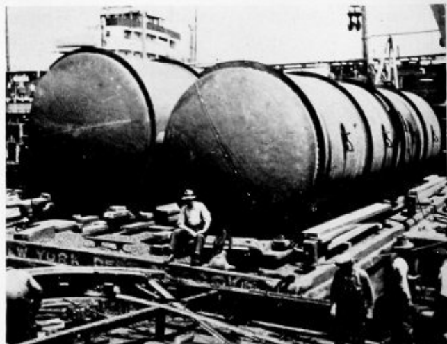
View of the finished pontoons
