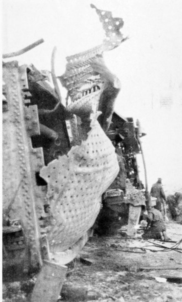
Fig. 3.—Two men were injured in this boiler explosion
