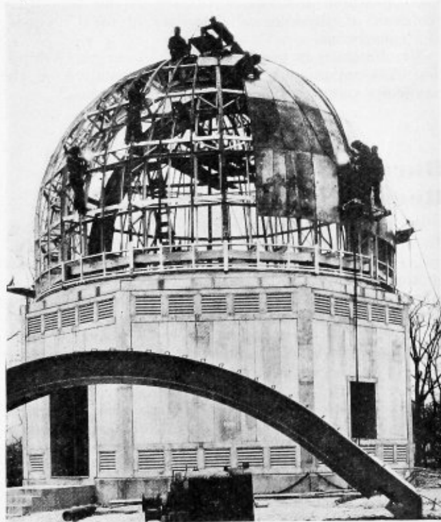
Construction of observatory dome
