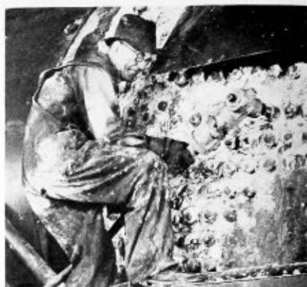
Hercules pneumatic wrench in service
