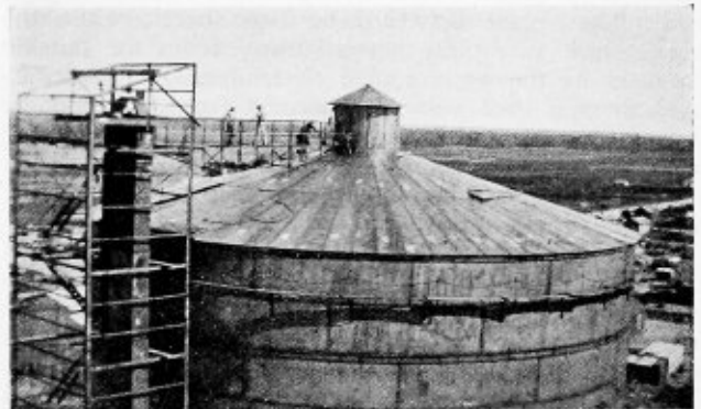
Fig. 6.—View of finished roof
