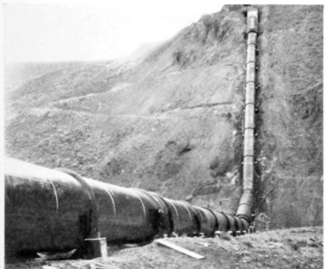
Fig. 2—Siphon 10 feet 6 inches in diameter
