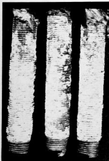
Door sheet staybolts as removed
