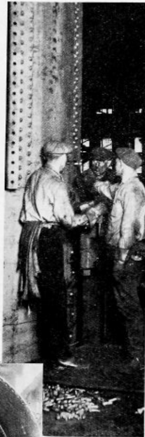
Fig. 6.—(Above) Hydraulic riveting with pure nickel rivets. Fig. 7.—(Left) Interior of tank car. Fig. 8.—(Below) Bevel shearing nickel-clad steel plate for tank car
