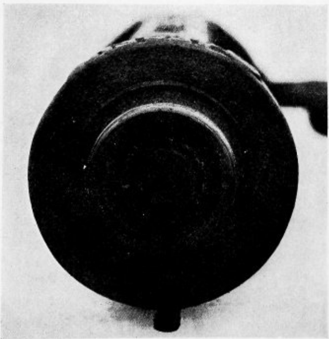
Fig. 6.—The clogged water glass which caused the crown-sheet failure shown above
