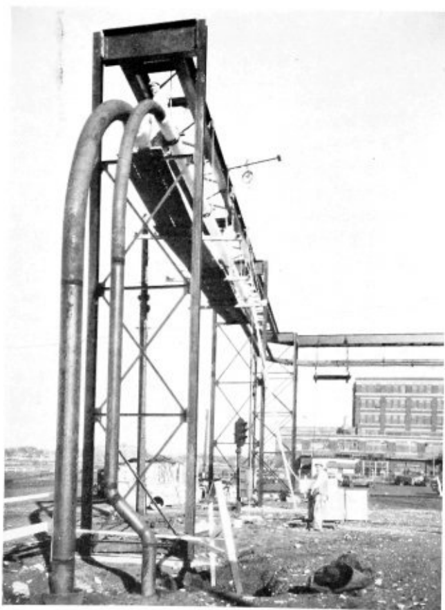
Where 18-inch steam line and 8-inch water return lines emerge from tunnel and are carried on bridge to steam distributing point
