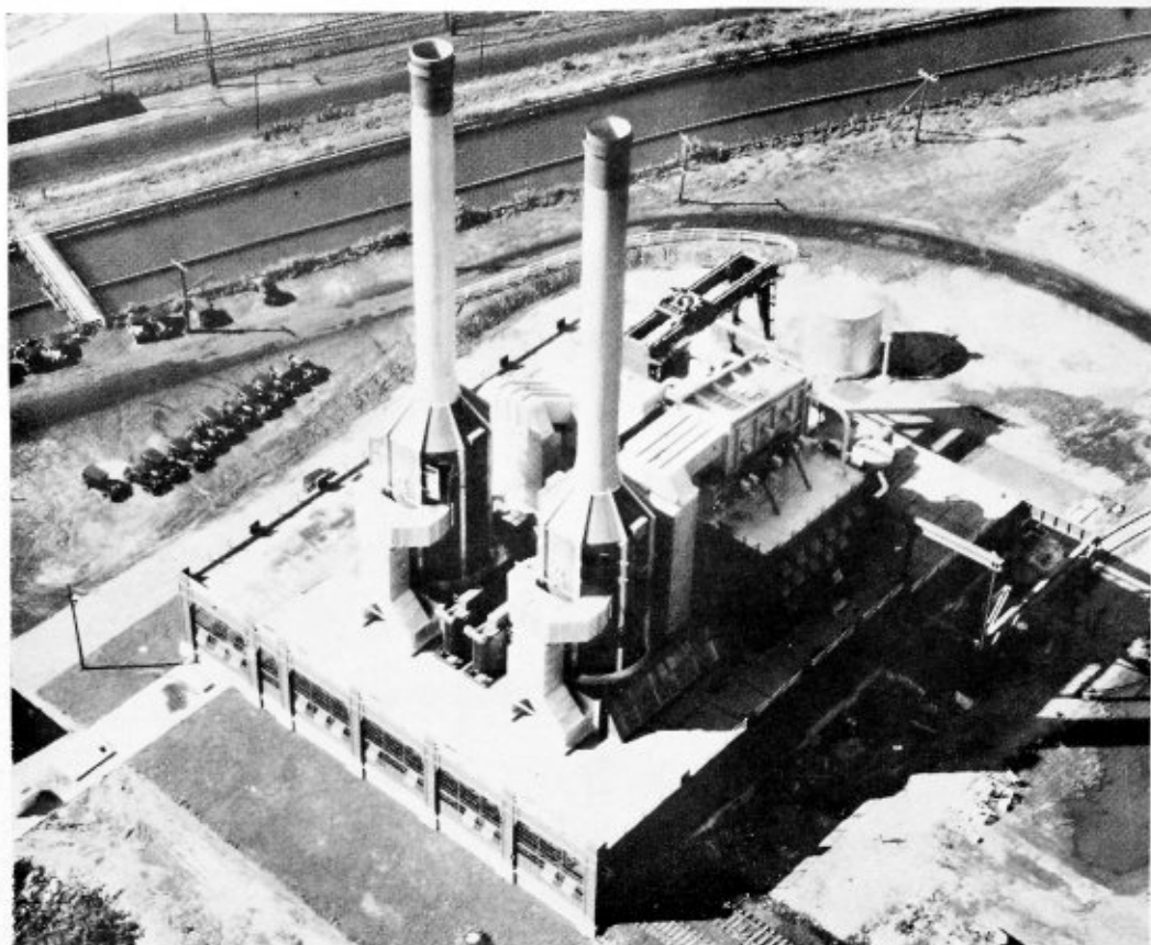
View from above northeast corner of General Electric mercury-steam- electric power plant
