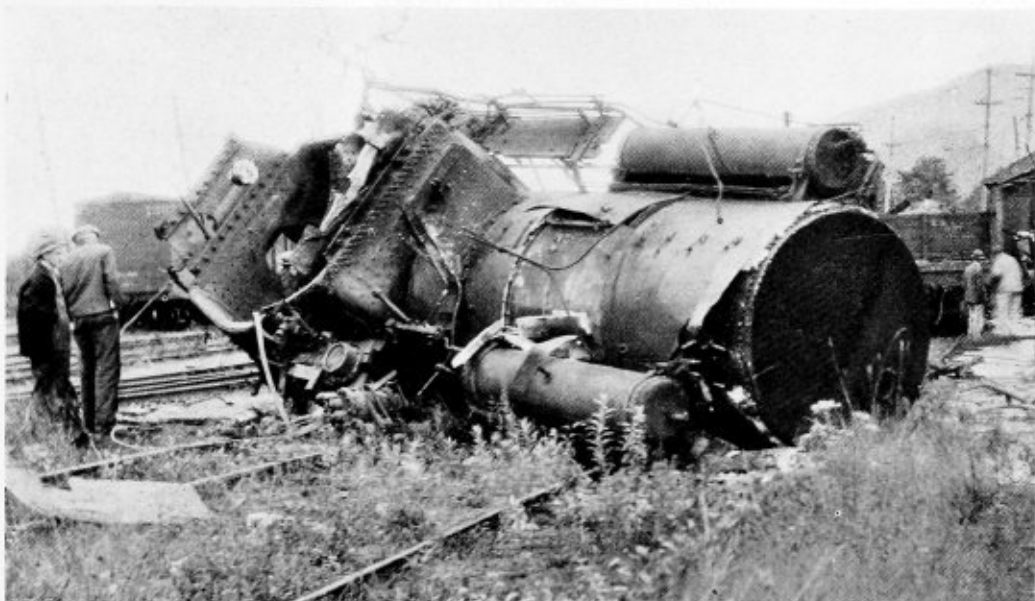
Fig. 3.—This low water failure resulted in the death of one railroad employee
