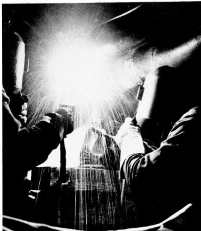
Welding high-pressure steam piping at River Rouge power plant
