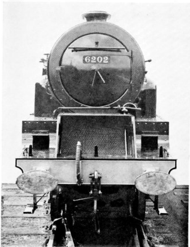
Front view showing oil-cooling radiator below the smokebox
