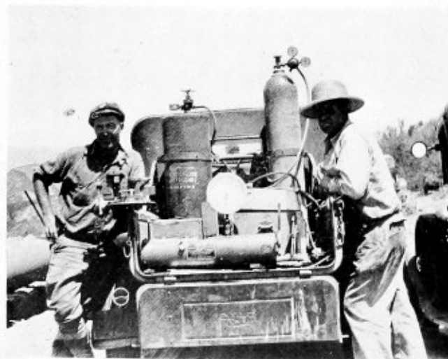
Fig. 2.—Field set for weld testing
