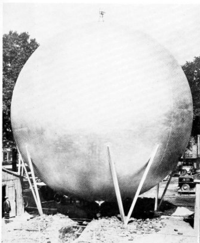
Horton-sphere, 36 feet in diameter
