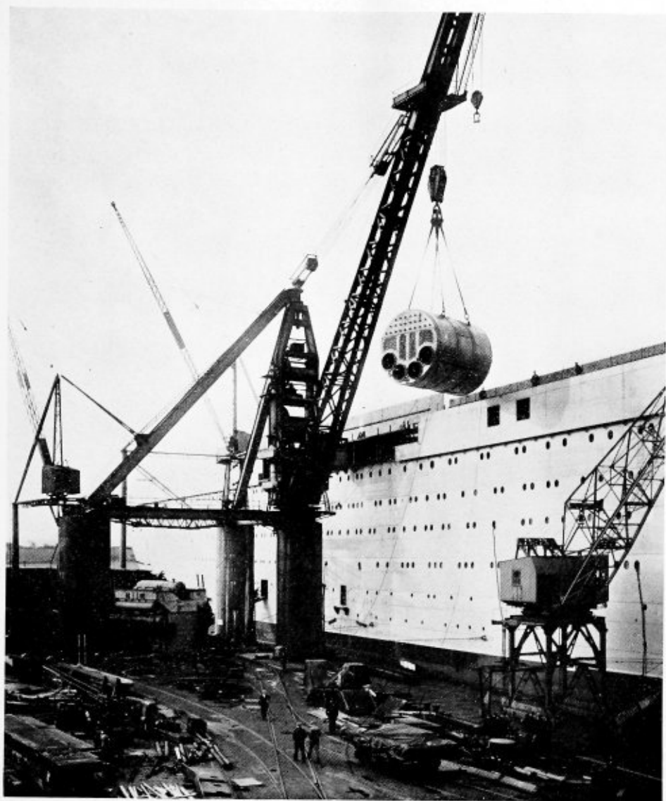
One of the auxiliary Scotch boilers being lowered into the ship
