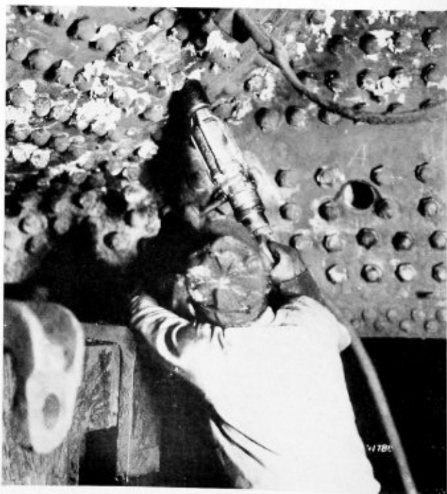
New wrench specially adapted to locomotive boiler work
