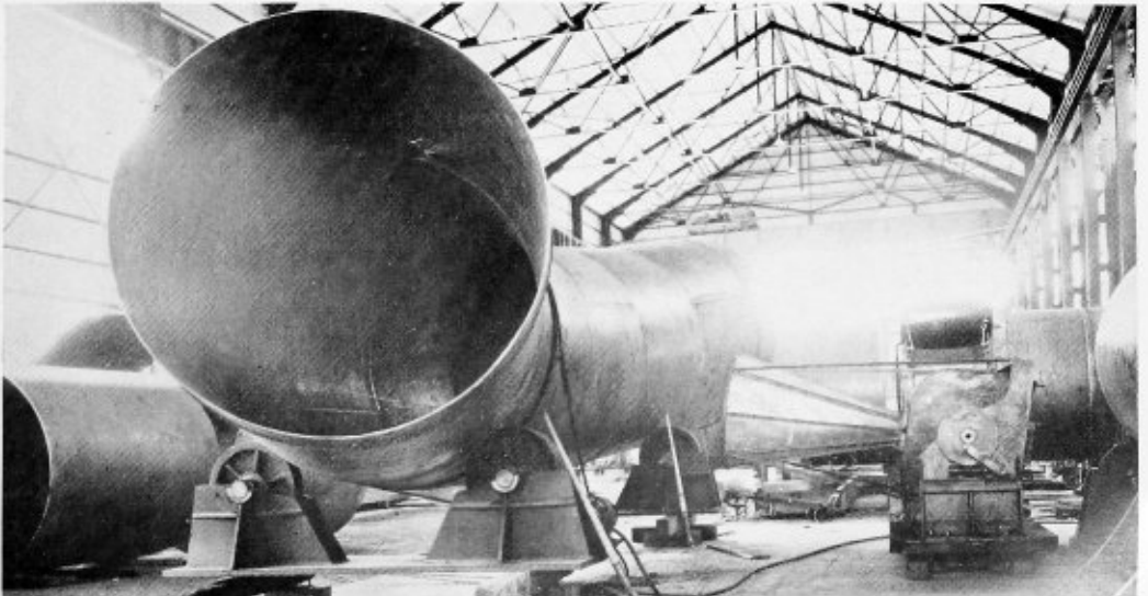
Fig. 11.—The same equipment, shown above, in use for the examination of a welded pipe section
