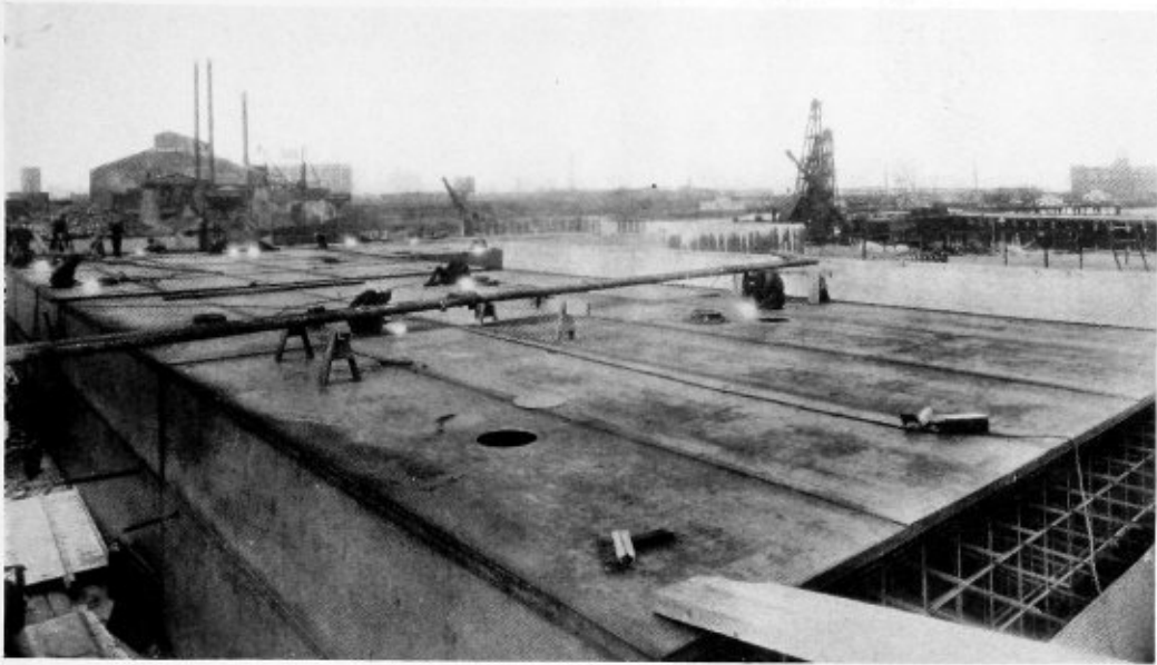
Fig. 1.—Arc-welding the roof plating of a 200,000 gallon rectangular bulk storage tank
