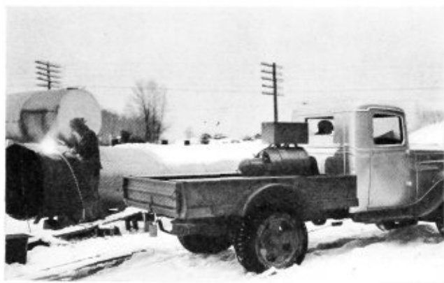
Motor truck fitted with power take-off driving arc-welding generator
