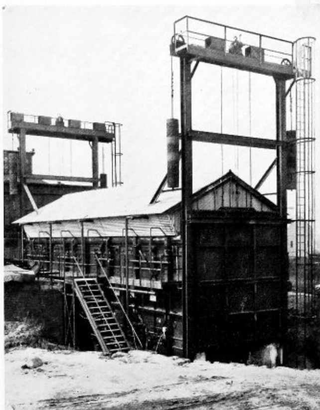
Exterior of gas-fired annealing furnace
