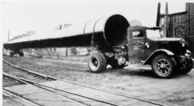
150-foot smoke stack being shipped to location
