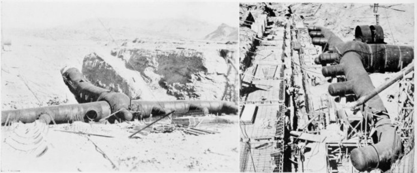
Giant welded inlet manifold for Colorado River Aqueduct
