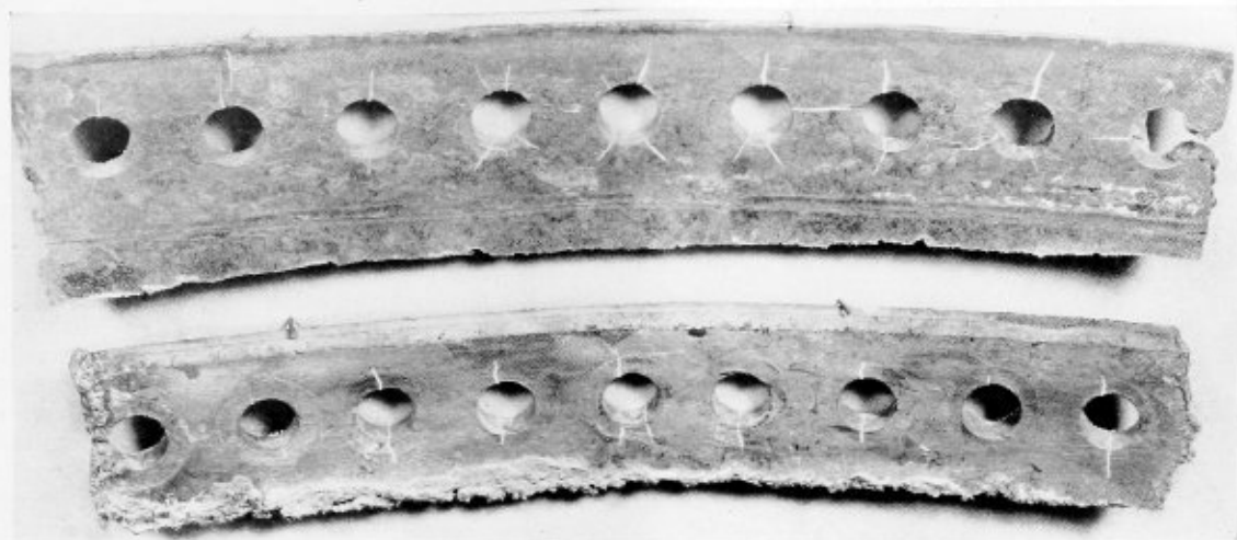
Fig. 2.—Typical examples of caustic-embrittlement cracks in girth seam of horizontal tubular boiler
