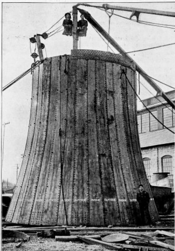
FIG. 12.—BELL SHAPED PORTION OF SELF-SUPPORTING STACK.
