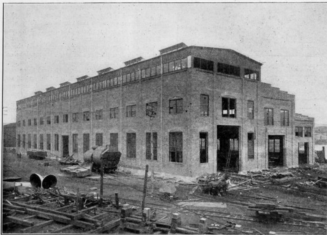
FIG. 4.—EXTERIOR OF THE COMPLETED SHOP.
