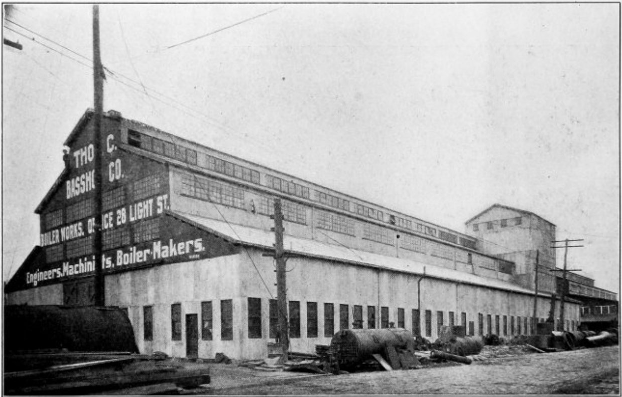
FIG. 2.—EXTERIOR VIEW OF BASSHOR BOILER SHOP, SHOWING THE LARGE BOOM DERRICK FOR UNLOADING MATERIAL.
