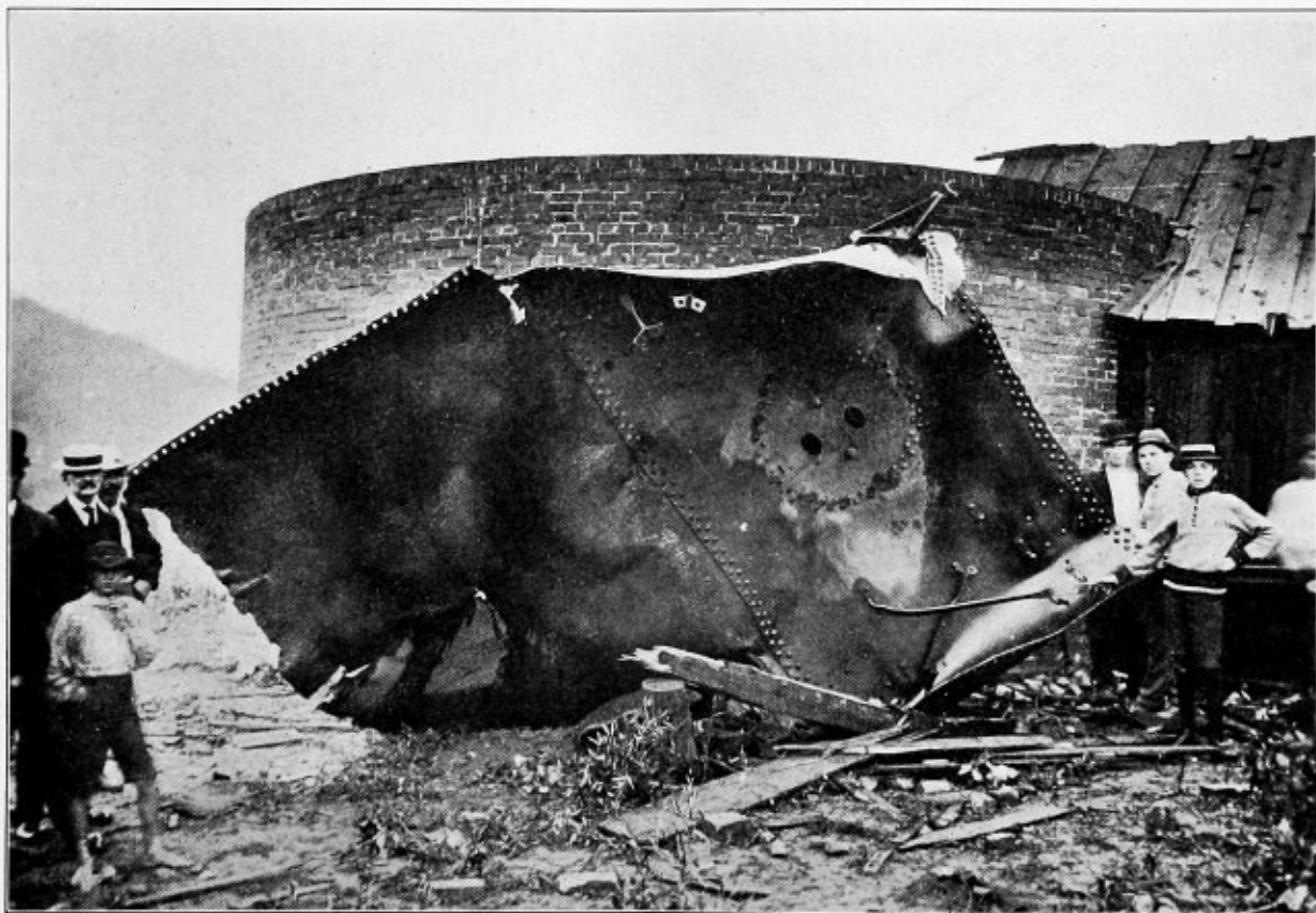
SECTION OF BOILER SHELL FROM EXPLODED BOILER AT MONONGAHELA CITY, PA.
