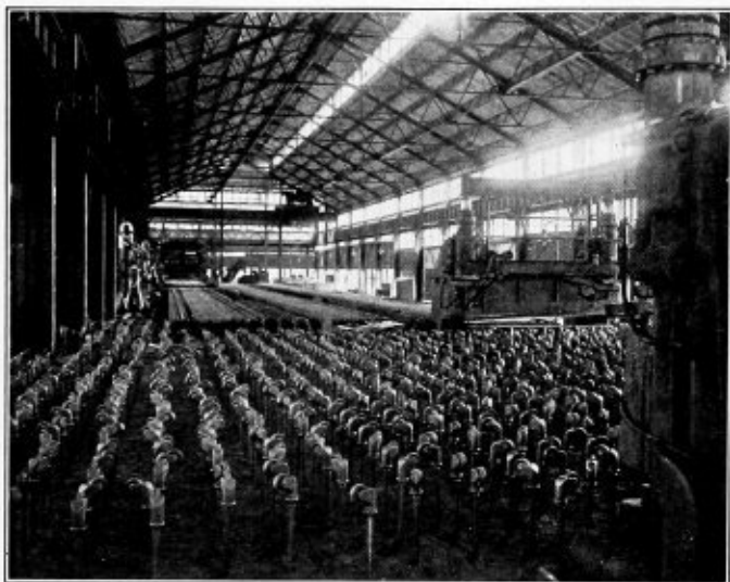
PLATE MILL, STRAIGHTENING ROLLS AND GUILLOTINE SHEARS AT WORTH BROS., COATESVILLE, PA.
