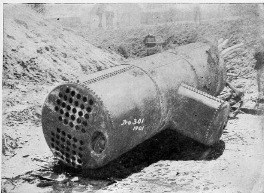
FIG. 6.—REAR END OF BOILER WHOSE EXPLOSION WAS DUE TO SCALE FORMATION.
