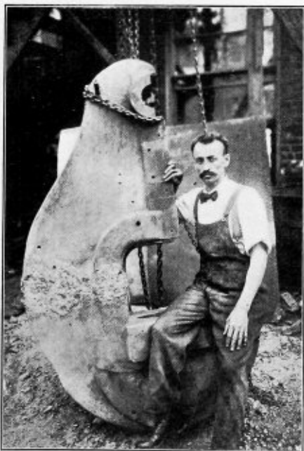
A SAMPLE OF HEAVY WORK WELDED BY THE OXY-ACETYLENE PROCESS.
