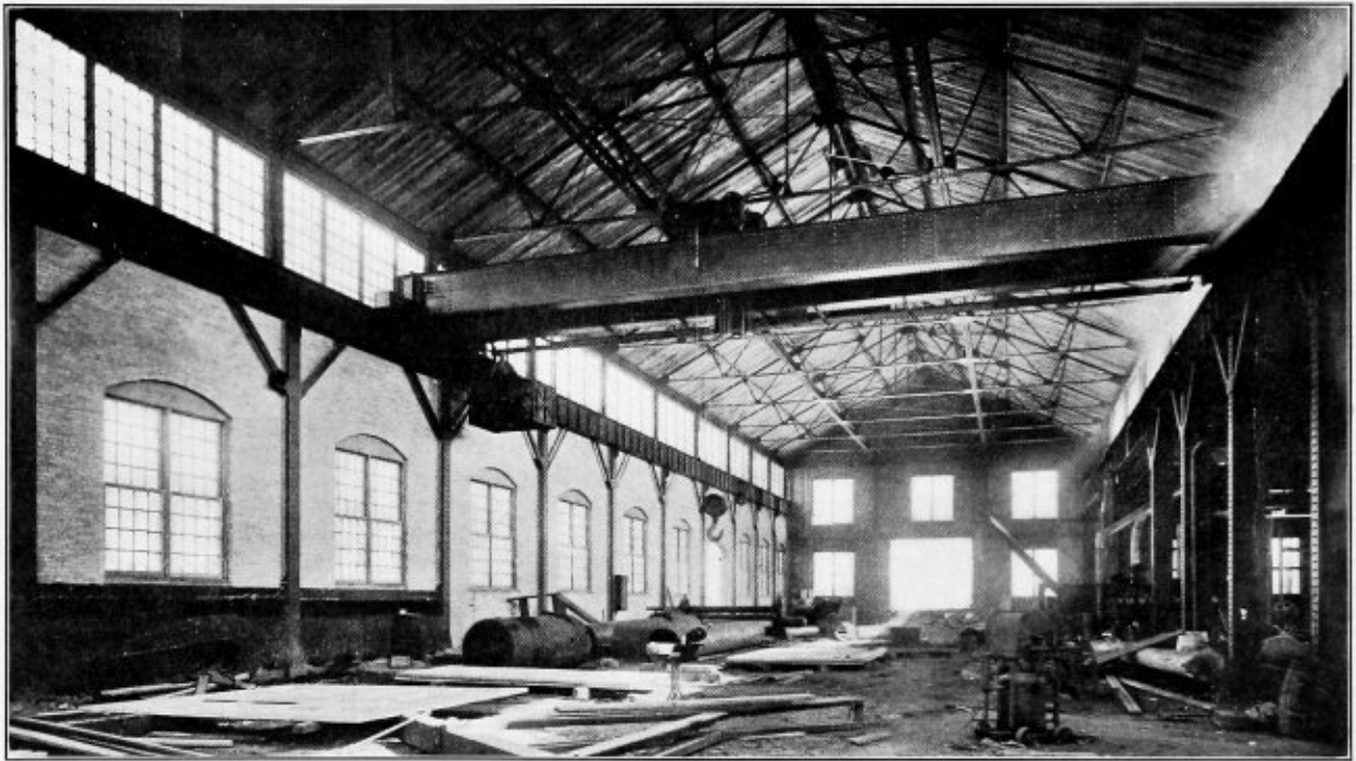
FIG. 5.—ERECTING FLOOR OF THE UNION BOILER WORKS, LOOKING EAST.
