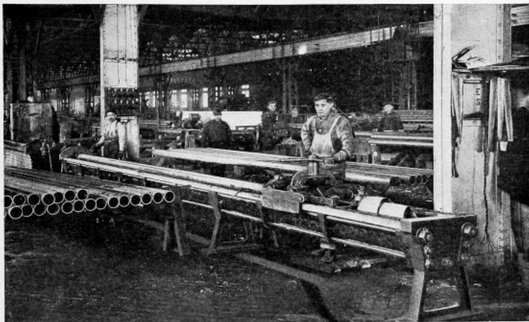
FIG. 4.—TESTING BOILER TUBES.
