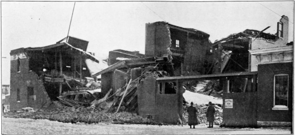
FIG. 2.—BUILDING WRECKED BY THE EXPLOSION.
