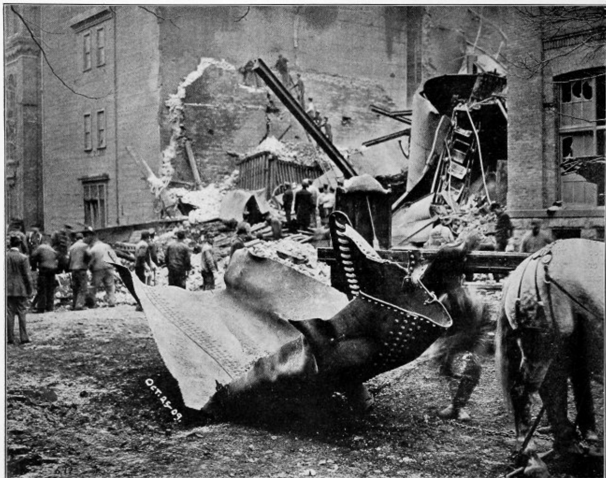
FIG. 2.—ONE OF THE SIX BURSTED STEAM DRUMS.
