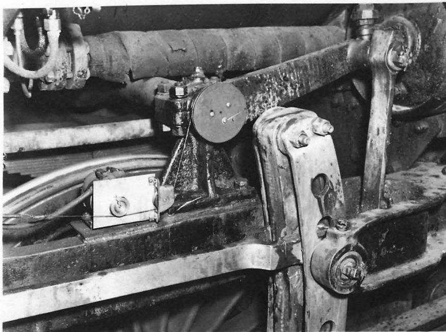
Cutoff position selsyn transmitter application to reverse shaft and transverse lever.
