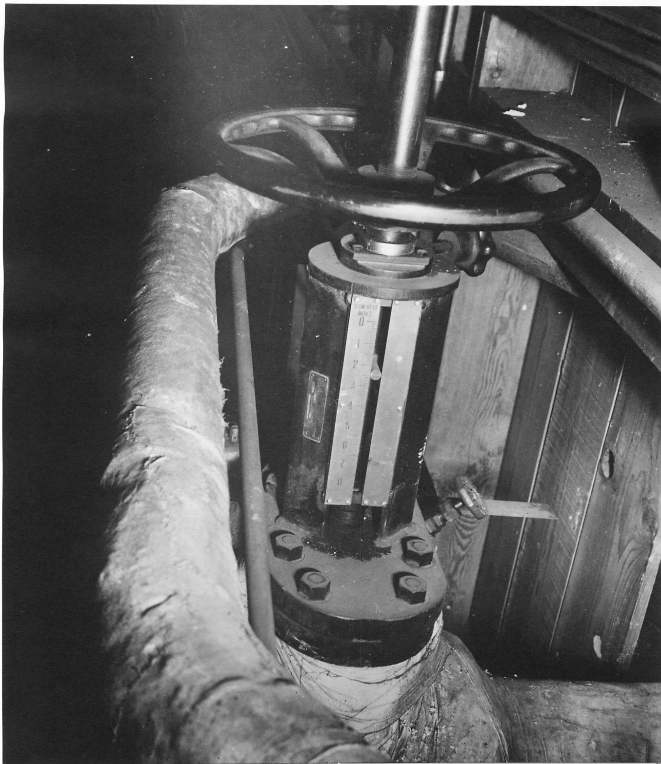
CLOSE-UP OF 8" ADJUSTABLE ORIFICE Showing hand wheel and segment height indicator, with vernier scale just under hand wheel.
